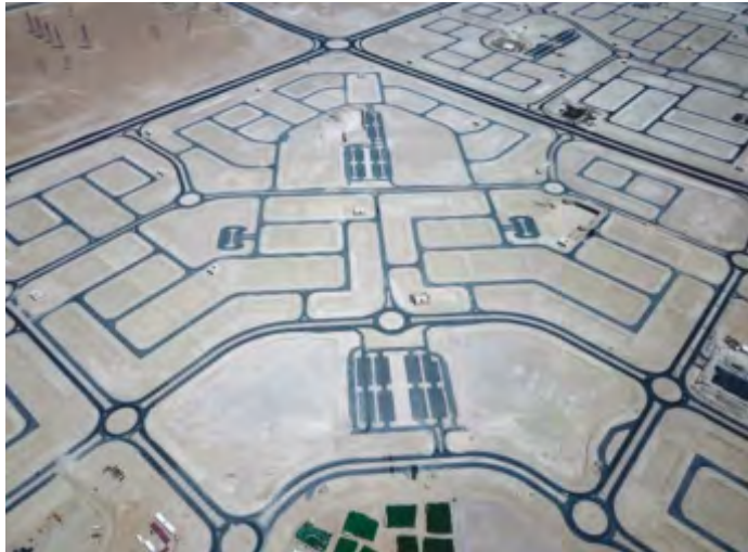
SOUTH AL MUTLAA (N1&N4) INFRASTRUCTURE WORKS-KUWAIT
