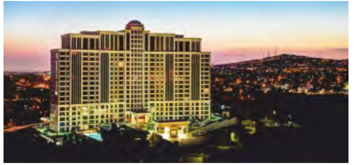
DELUXIA ATAŞEHİR ELECTRICAL WORKS, İSTANBUL-TÜRKİYE
