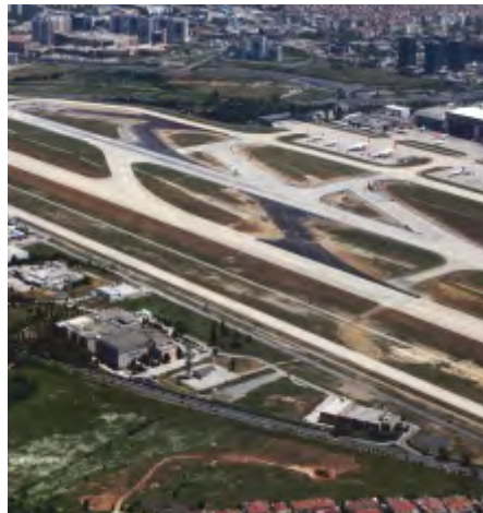
ATATÜRK AIRPORT RUNWAY-APRON-TAXIWAY İSTANBUL-TÜRKİYE
