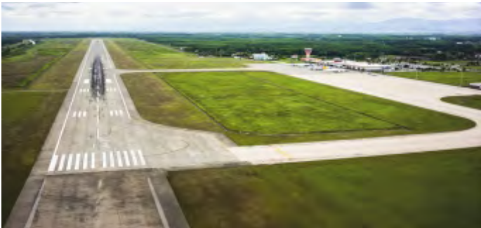
SAMSUN AIRPORT, RUNWAY, TAXIWAY AND APRON REFURBISHMENT-TÜRKİYE
