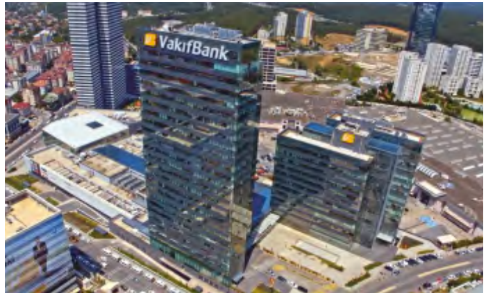
SERVICE BUILDING OF VAKIFLAR BANK GENERAL DIRECTORATE, ÜMRANİYE, İSTANBUL-TÜRKİYE
