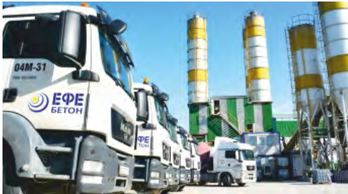
EFE BETON, CONCRETE BATCH PLANT FACILITY, LVIV-UKRAINE
