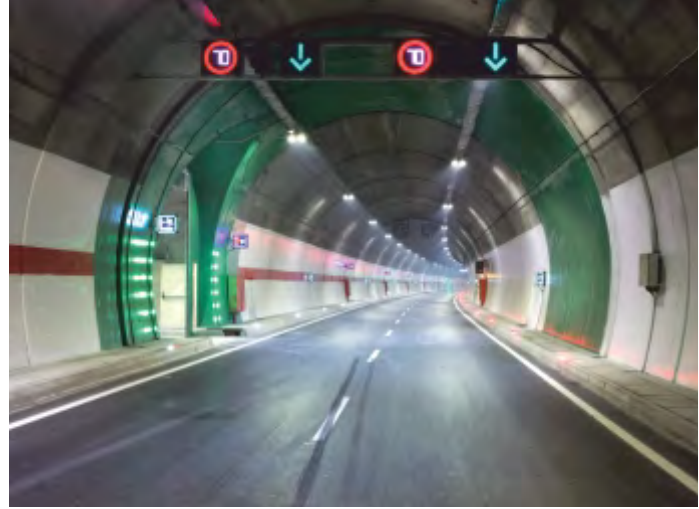
ZİGANA TUNNEL, TRABZON-TÜRKİYE
