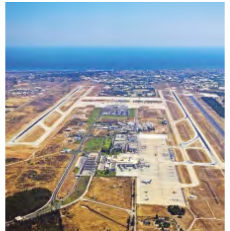
ANTALYA AIRPORT PAT SITES AND REPAIR WORKS-TÜRKİYE
