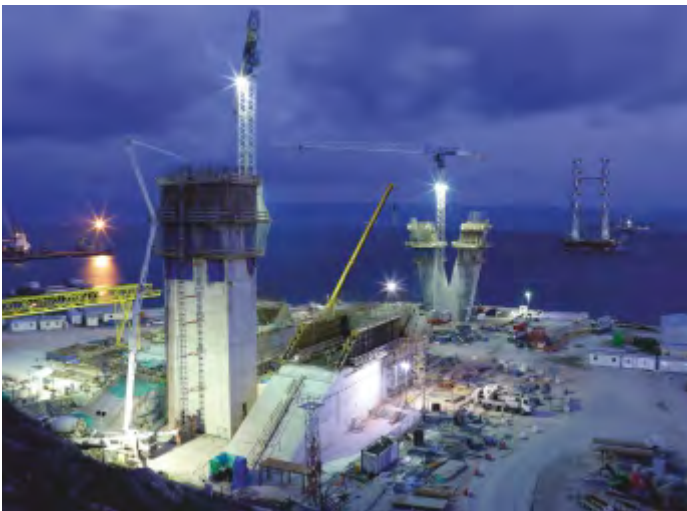
OSMAN GAZİ SUSPENSION BRIDGE, KOCAELİ-TÜRKİYE
