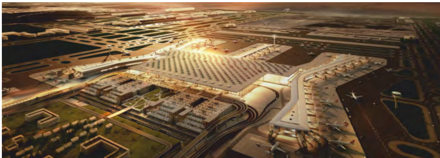
ISTANBUL AIRPORT PROJECT, PHASE I-TÜRKİYE
