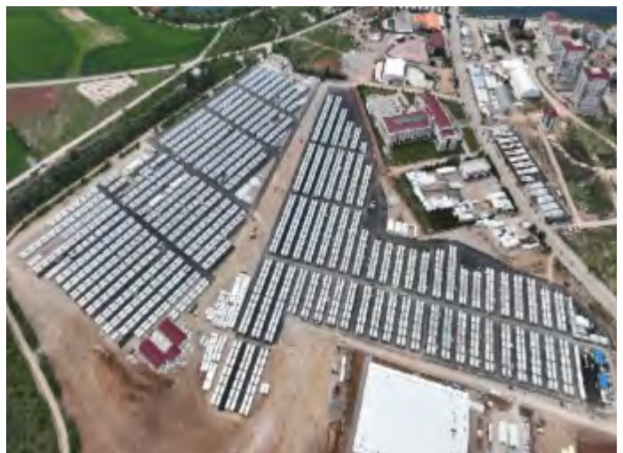
CONTAINER VILLAGES FOR EMERGENCY ACCOMMODATION (10 DIFFERENT CITIES)-TÜRKİYE
