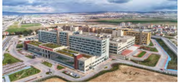
ESKİŞEHİR CITY HOSPITAL-TÜRKİYE
