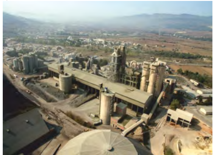
BOLU CEMENT PLANT CAPACITY INCREASE-TÜRKİYE
