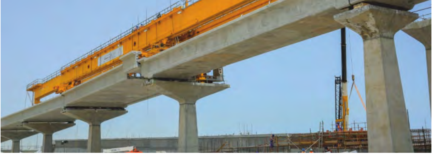
DOHA METRO RED LINE SOUTH ELEVATED AND AT GRADE-QATAR
