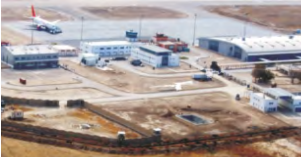
AIRPORT TERMINAL AND SERVICE BUILDINGS, MAZAR-E-SHARIF-AFGHANISTAN
