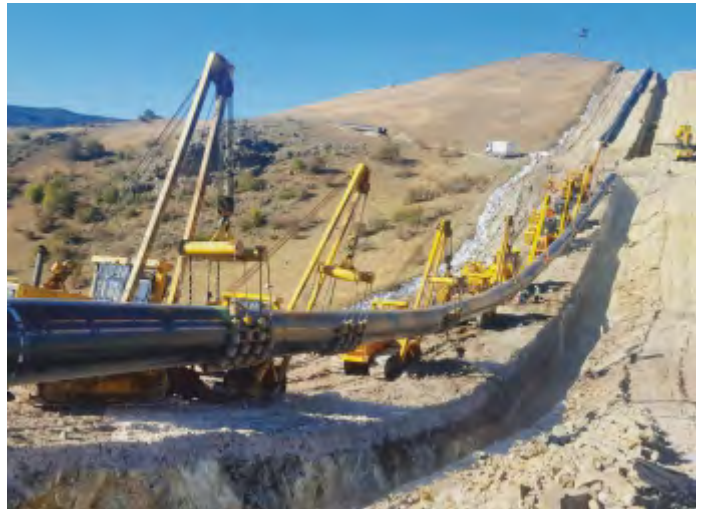
POSOF-ERZİNCAN TRANS ANATOLIAN NATURAL GAS PIPELINE-TÜRKİYE
