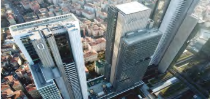
QUASAR İSTANBUL ELECTRICAL WORKS, İSTANBUL-TÜRKİYE
