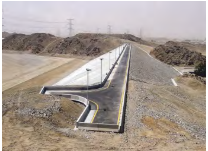
STORM WATER DRAINAGE AND DAMS, JEDDAH-SAUDI ARABIA
