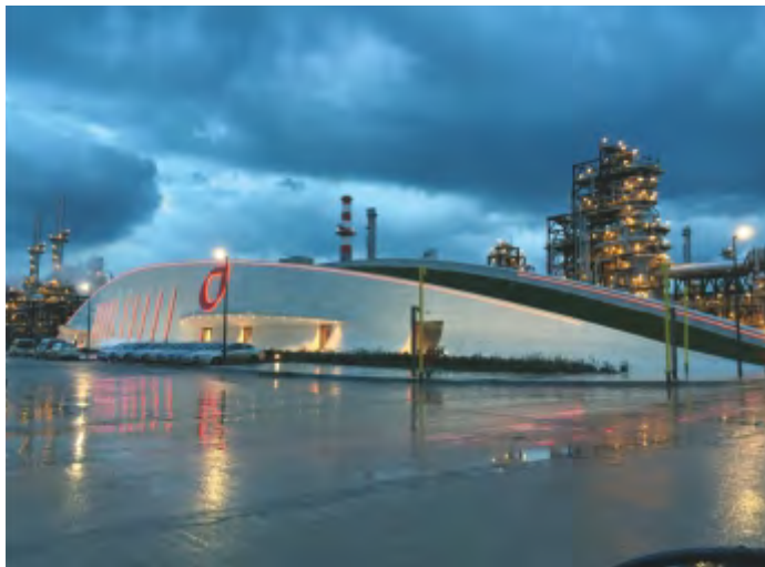
THE TURKISH PETROLEUM REFINERIES CORPORATION RUP PROJECT MAIN CONTROL BUILDING KOCAELI-TÜRKİYE
