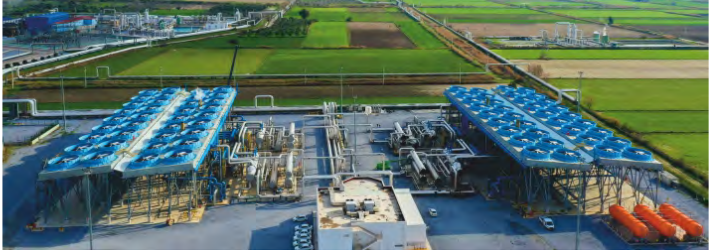
EFELER GEOTHERMAL POWER PLANT, AYDIN-TÜRKİYE
