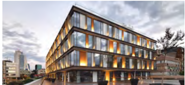
RÖNESANSBİZ MECİDİYEKÖY ELECTRICAL WORKS, İSTANBUL-TÜRKİYE
