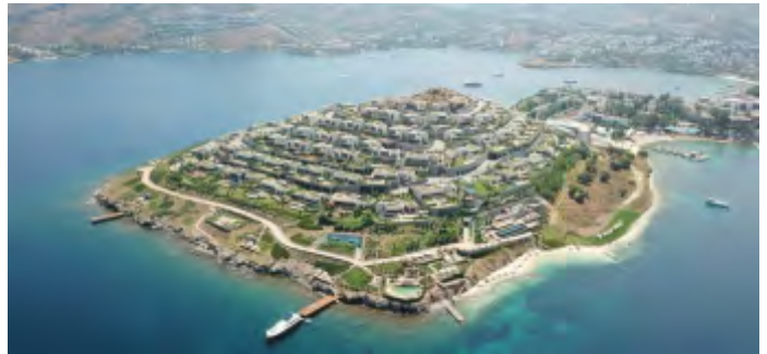
THE RITZ-CARLTON RESIDENCES BODRUM ELECTRICAL WORKS, MUĞLA-TÜRKİYE
