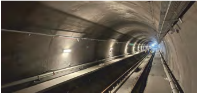
MECİDİYEKÖY-MAHMUTBEY METRO LINE ELECTRICAL WORKS, İSTANBUL-TÜRKİYE
