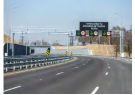
CONSTRUCTION AND OPERATION OF THE MOTOR ROAD BIG ALMATY RING ROAD (BAKAD), ALMATY-KAZAKHSTAN
