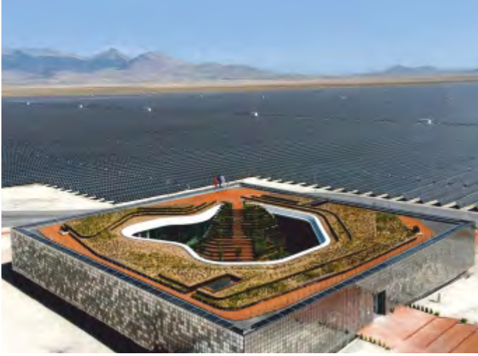
KALYON KARAPINAR SOLAR POWER PLANT, KONYA-TÜRKİYE
