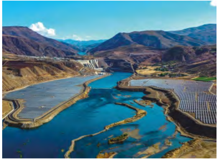
LOWER KALEKÖY DAM AND HEPP, BİNGÖL-TÜRKİYE
