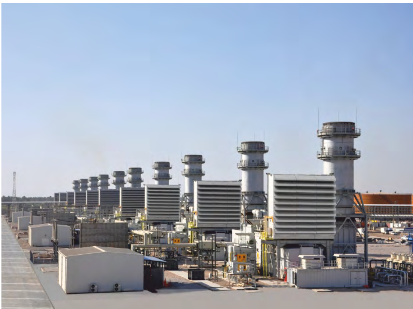
AL-KHAIRAT SIMPLE CYCLE POWER PLANT-IRAQ
