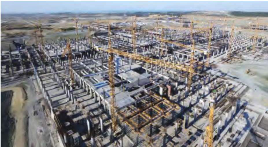
İSTANBUL AIRPORT (PRODUCTION AND INSTALLATION OF DOUBLE TEE FLOORING ELEMENTS)-TÜRKİYE
