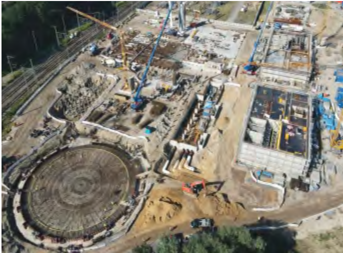
CIVIL WORKS OF DRADENAU CHP-PLANT, HAMBURG-GERMANY
