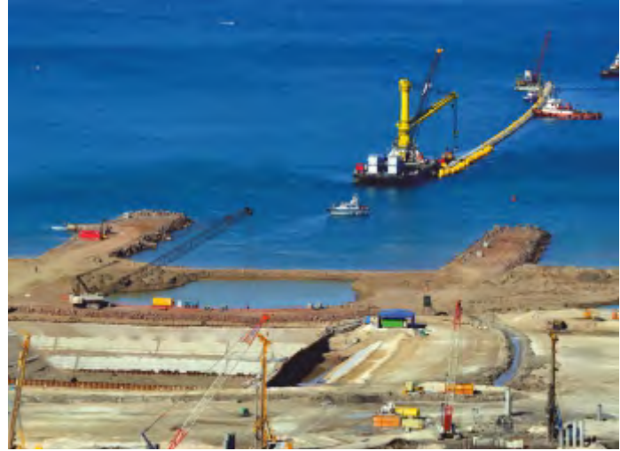
MARINE WORKS of MOSTAGANEM COMBINED CYCLE POWER PLANT-ALGERIA
