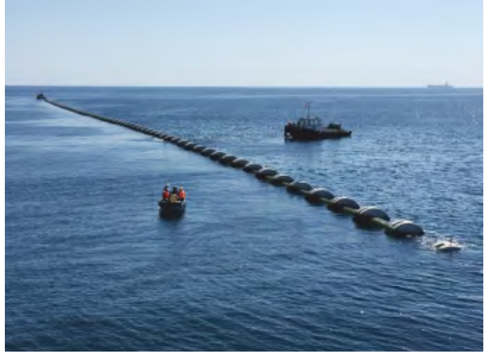
SALALAH WASTEWATER SYSTEM MARINE OUTFALL-OMAN
