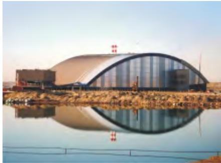
BAKU WASTE-TO-ENERGY PLANT-AZERBAIJAN
