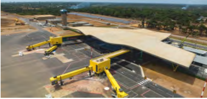
FREETOWN INTERNATIONAL AIRPORT-SIERRA LEONE
