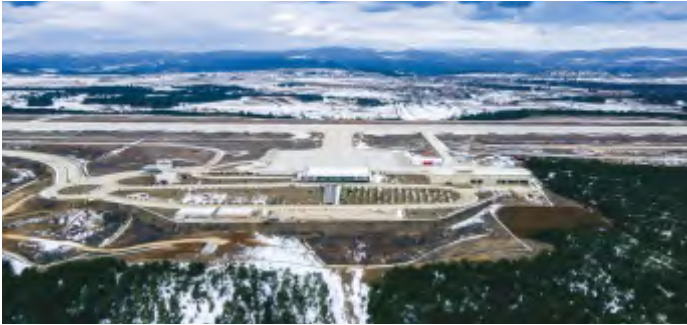
KASTAMONU AIRPORT, RUNWAY, TAXIWAY AND APRON REFURBISHMENT-TÜRKİYE
