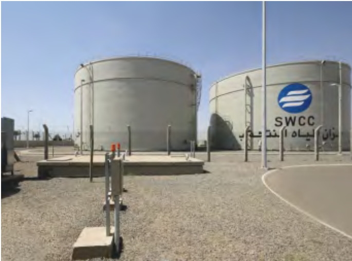
SHUQAIQ POTABLE WATER PIPELINE PHASE II-SAUDI ARABIA
