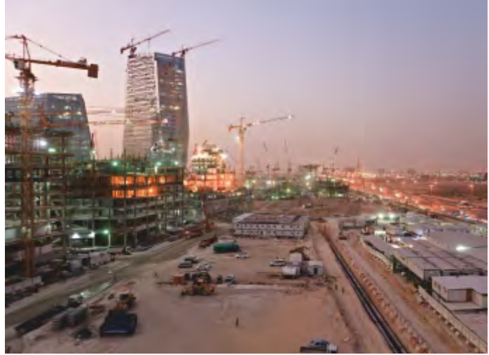
KAFD KING ABDULLAH FINANCIAL DISTRICT INFRASTRUCTURE, RIYADH-SAUDI ARABIA
