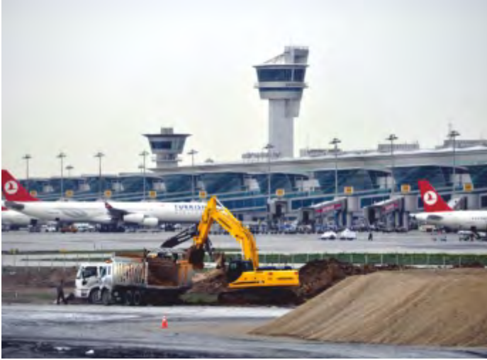
ATATÜRK AIRPORT RUNWAY RENOVATION, İSTANBUL-TÜRKİYE
