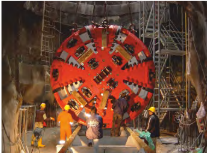
BALTALİMANI WASTE WATER TUNNEL, İSTANBUL-TÜRKİYE
