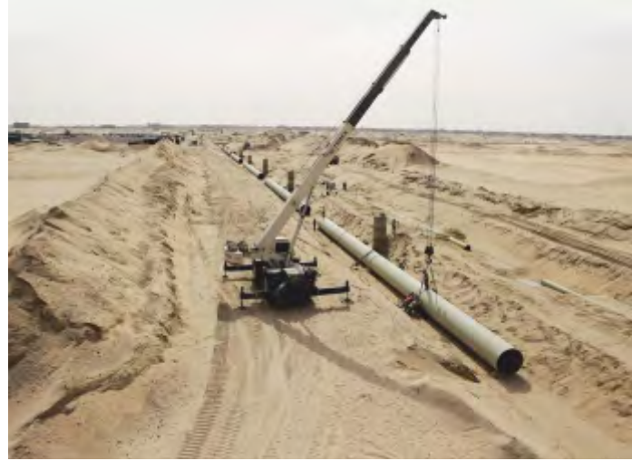
DAMMAM NORTH HOUSING PROGRAM INFRASTRUCTURE WORKS-SAUDI ARABIA
