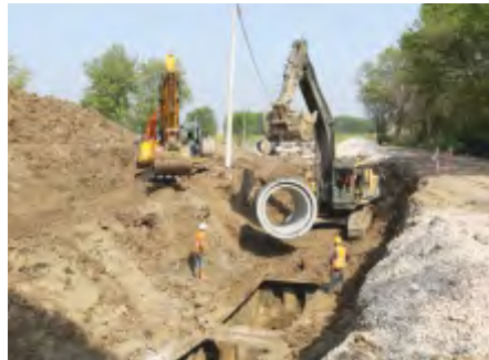
BUSKİ OVAAKÇA-HASANAĞA SEWAGE COLLECTOR LINES BURSA-TÜRKİYE
