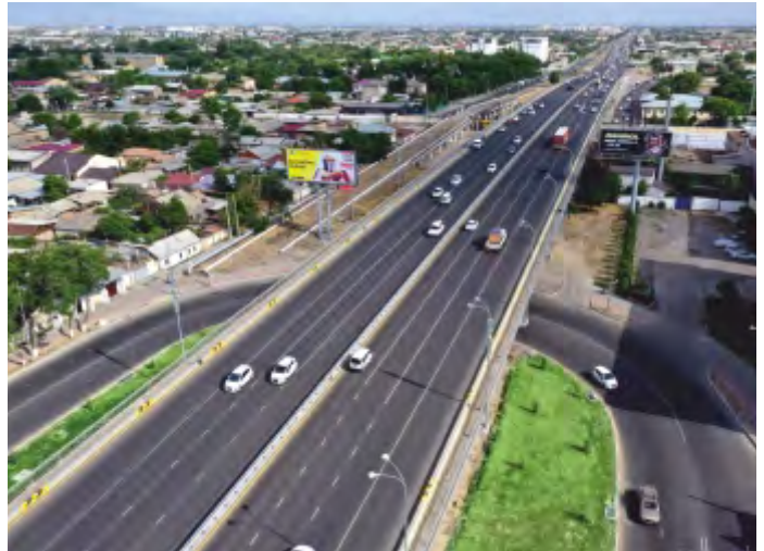
ROAD AND BRIDGE, TASHKENT-UZBEKISTAN
