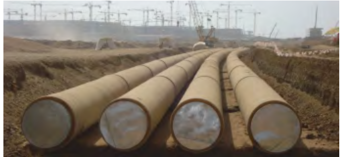
KING ABDULLAH SCIENCE AND TECHNOLOGY UNIVERSITY (KAUST) INFRASTRUCTURE WORKS THUWAL-SAUDI ARABIA
