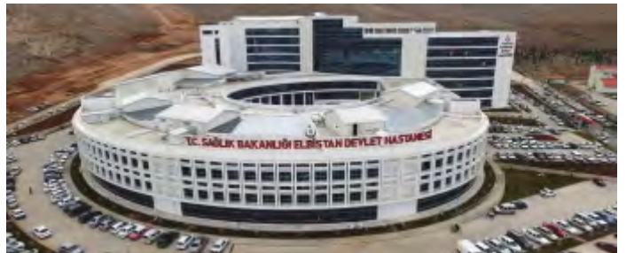
ELBİSTAN STATE HOSPITAL REVISED ADDITIONAL BUILDING (300 BED), KAHRAMANMARAŞ-TÜRKİYE
