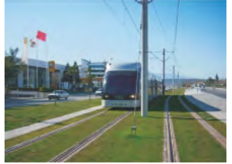
LIGHT RAIL SYSTEM 1st PHASE CONSTRUCTION WORKS ANTALYA-TÜRKİYE
