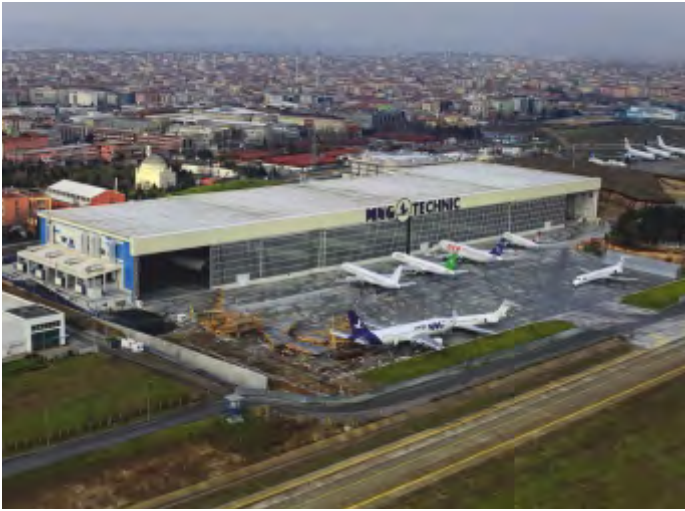
AIRCRAFT MAINTENANCE HANGAR, İSTANBUL-TÜRKİYE
