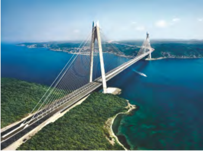
THIRD BOSPHORUS BRIDGE AND NORTHERN MARMARA MOTORWAY, İSTANBUL-TÜRKİYE
