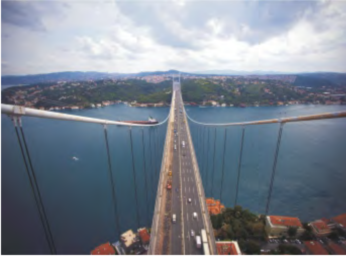
FATİH SULTAN MEHMET BRIDGE-PAVEMENT REHABILITATION, İSTANBUL-TÜRKİYE
