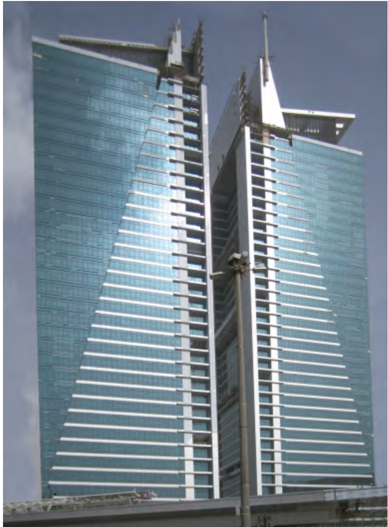
OLAYA TOWERS, RIYADH-SAUDI ARABIA
