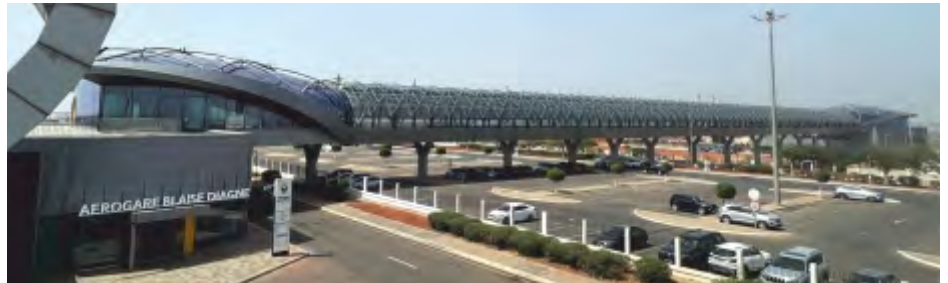
TER AIBD STATION, DAKAR-SENEGAL
