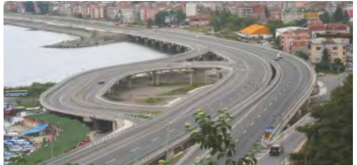
BLACK SEA COASTAL ROAD ÇARŞIBAŞI-TRABZON-ARAKLI AND TRABZON-MAÇKA SEGMENT TÜRKİYE
