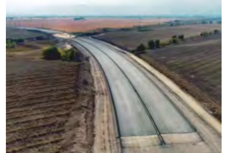
DESIGN AND EXECUTION OF LOT 1 & LOT 2 RING MOTORWAY BUCHAREST-ROMANIA
