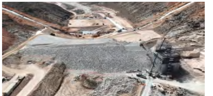
FLOOD PROTECTION DAM AT WADI ADAWNIB, SALALAH-OMAN
