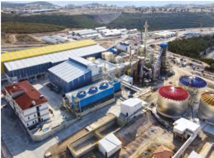
ETİMAĐEN EMET SULPHURIC ACID PLANT (350.000 TON/YEAR), KÜTAHYA-TÜRKİYE
