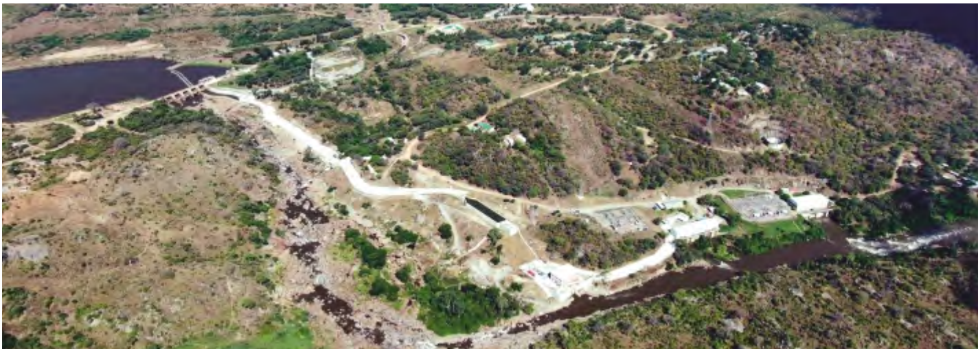
TEDZANI ELECTRICITY HYDROPOWER STATION EXPANSION-MALAWI
