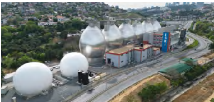
İSKİ BALTALIMANI BIOLOGICAL WASTEWATER TREATMENT PLANT, İSTANBUL-TÜRKİYE
