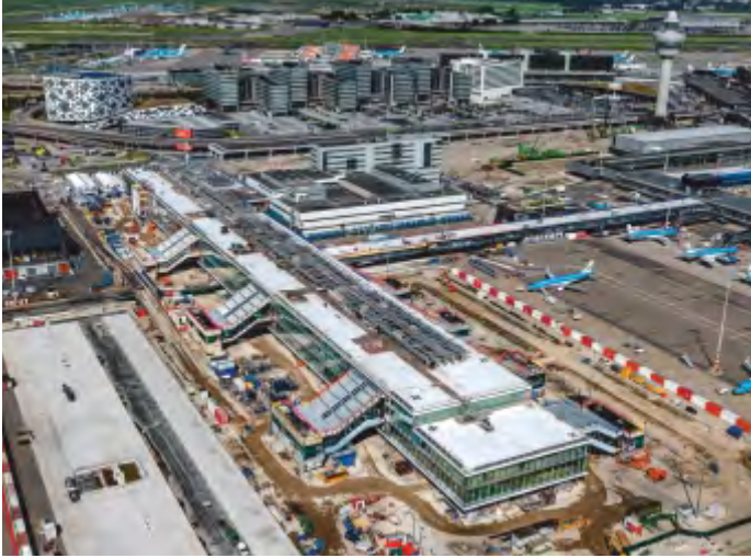
AMSTERDAM AIRPORT SCHIPHOL PIER A-NETHERLANDS
