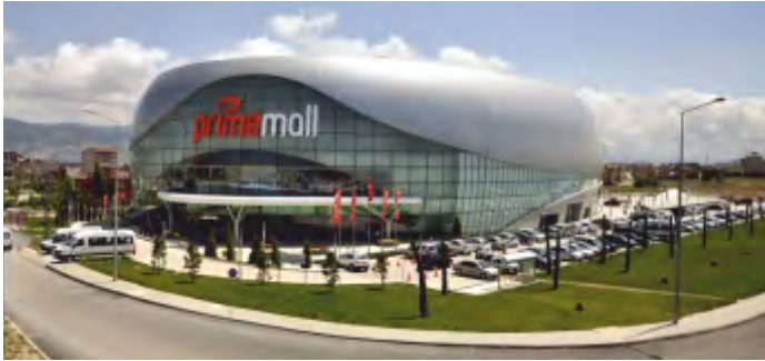
PRIME MALL ANTAKYA ELECTRICAL WORKS, HATAY-TÜRKİYE
