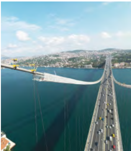
BOSPHORUS AND FATİH SULTAN MEHMET BRIDGES STRUCTURAL REINFORCEMENT / REPAIR, İSTANBUL-TÜRKİYE
