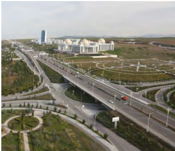
ARCABIL MOTORWAY, ASHGABAT-TURKMENISTAN
