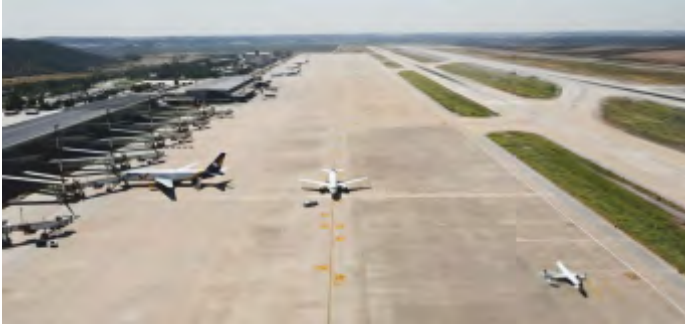
BODRUM MİLAS AIRPORT, RUNWAY, APRON, TAXIWAY, HELIPAD CONSTRUCTION, MUĞLA-TÜRKİYE
