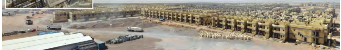
HOUSING COMPLEX AND SOCIAL FACILITIES (1416 VILLAS), BASRAH-IRAQ
