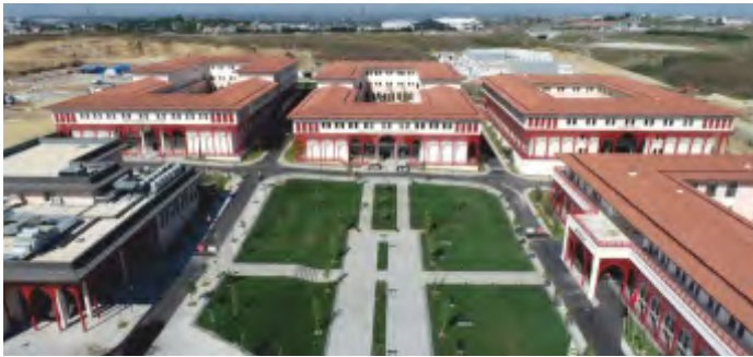
İBN HALDUN UNIVERSITY ELECTRICAL WORKS, İSTANBUL-TÜRKİYE
