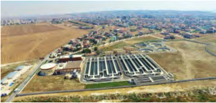
İSKİ SİLİVRİ ADVANCED BIOLOGICAL WASTEWATER TREATMENT PLANT, İSTANBUL-TÜRKİYE
