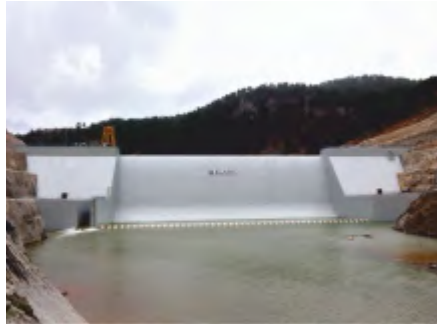
KARAKUZ DAM AND HEPP, ADANA-TÜRKİYE
