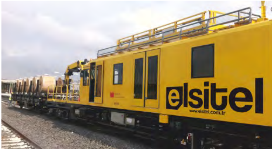
ANKARA-İSTANBUL HIGH SPEED TRAIN LINE PHASE 2, CABLING WORKS, İNÖNÜ-KÖSEKÖY-TÜRKİYE
