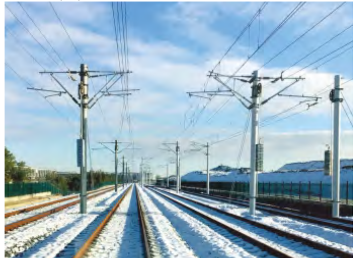
GAZIRAY HIGH SPEED TRAIN AND COMMUTER LINE, CATENARY SYSTEM, GAZİANTEP-TÜRKİYE
