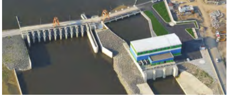
HYDROELECTRIC POWER PLANT, SAKARYA-TÜRKİYE
