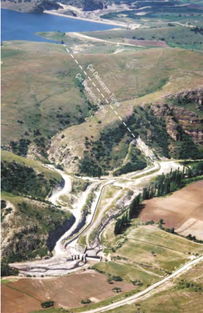
SARAYÖZÜ DAM AND ÇAT STREAM DIVERSION, AMASYA-TÜRKİYE
