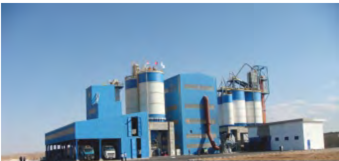
GÜRİŞ RAQQA KLINKER MILLING PLANT, RAKKA-SYRIA
