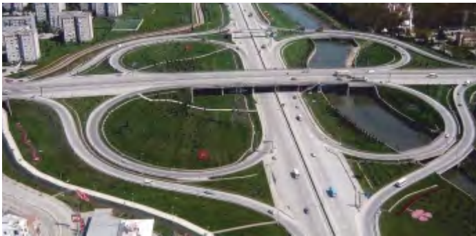
BALIKESİR DURSUNBEY INTERCHANGE AND UNDERPASS BRIDGE (12 KM HIGHWAY AND 7 BRIDGES)-TÜRKİYE
