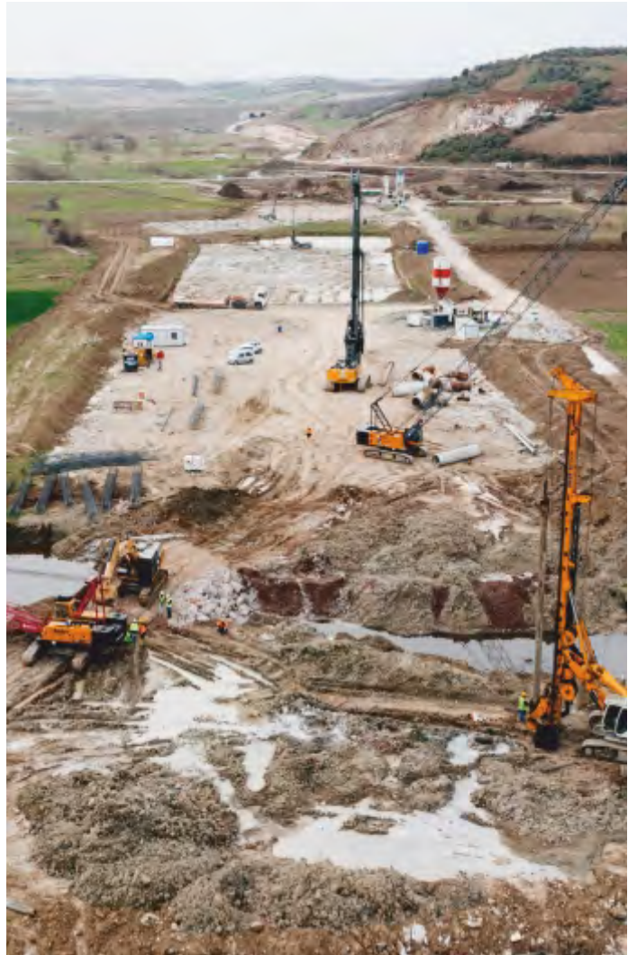
ZEYTİNBAĞI PROVINCIAL ROAD (BURSA-KARACABEY SECTION) AND TEKNOSAB INTERCHANGE TÜRKİYE
