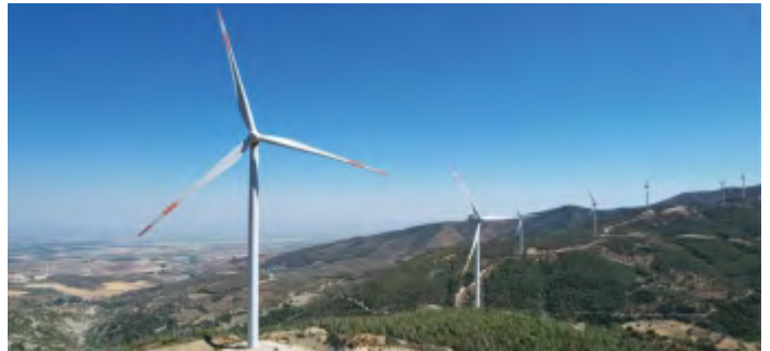
ÇERÇİKAYA-ŞENBÜK WPP (WIND POWER PLANT-114 MW), HATAY-TÜRKİYE
