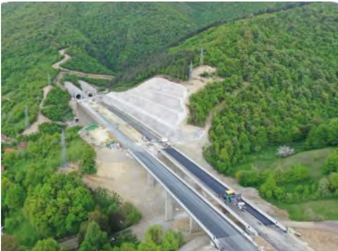
5C CORRIDOR HIGHWAY ZENICA TUNNEL-BOSNIA AND HERZEGOVINA
