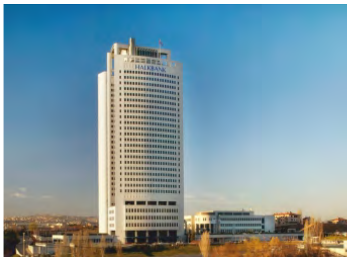
HALKBANK HEADQUARTERS BUILDING, ANKARA-TÜRKİYE
