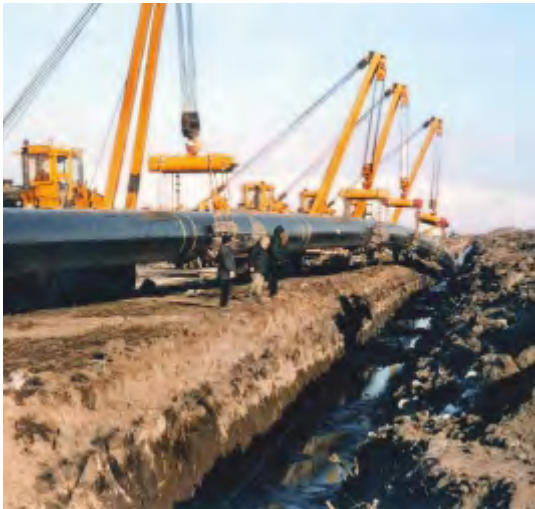
ERZURUM-İMRANLI (SİVAS) NATURAL GAS PIPELINE, ERZURUM-TÜRKİYE
