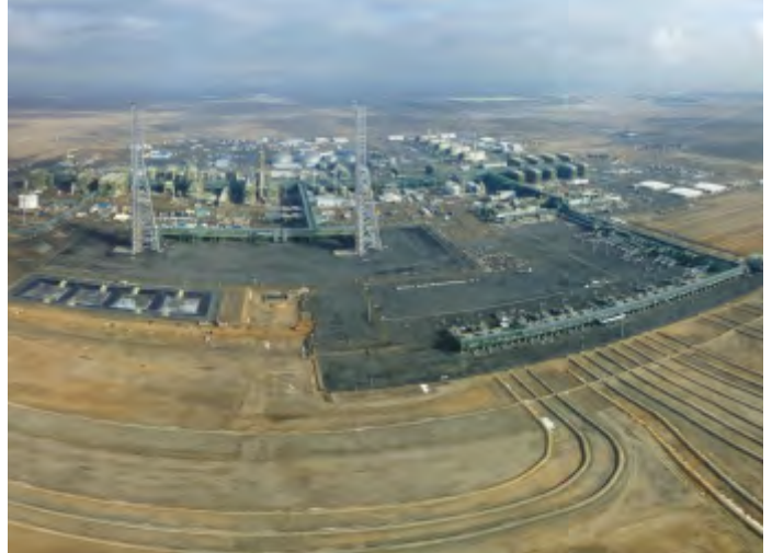
FGP 3GP MECHANICAL, ELECTRICAL AND INSTRUMENTATION INSTALLATION WORKS TENGİZ-KAZAKHSTAN
