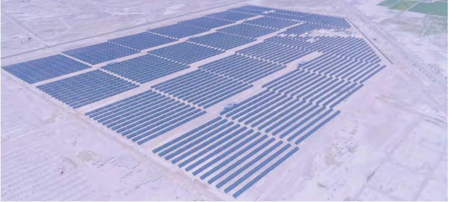
POWER PLANT (15 MW), KANDAHAR-AFGHANISTAN
