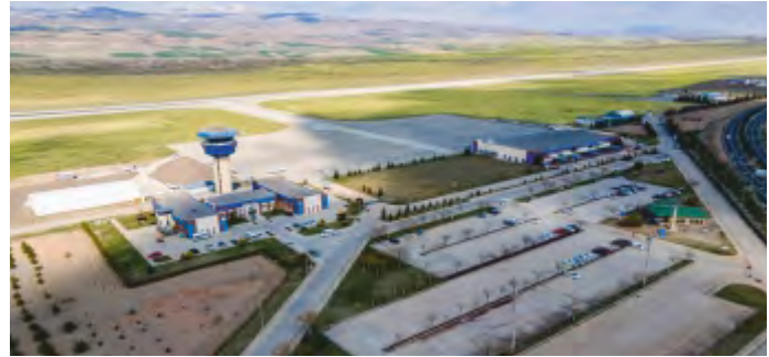
KAPADOKYA AIRPORT, RUNWAY, TAXIWAY AND APRON REFURBISHMENT-TÜRKİYE
