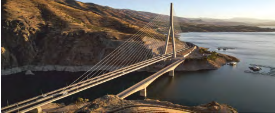
KÖMÜRHAN CABLE STAYED BRIDGE AND TUNNELS, ELAZIĞ-TÜRKİYE
