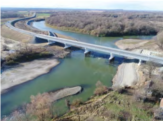
STRYI-TERNOPIL-KROPYVNYTSKYI-ZNAMIANKA ROAD (M-30) DNIESTER RIVER BRIDGE UKRAINE
