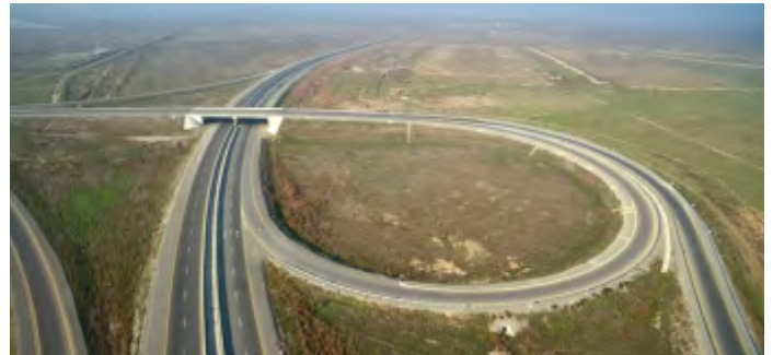
HACIKABUL-KURDEMİR ROAD REHABILITATION-AZERBAIJAN
