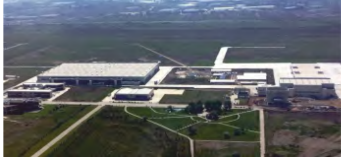
TAI HELICOPTER MANUFACTURING AND TEST FACILITIES, ANKARA-TÜRKİYE
