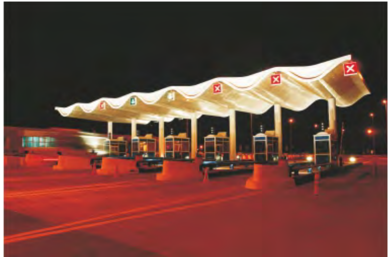
TANGER-PORT QUED R'MEL MOTORWAY, TANGER RN2 SECTION-MOROCCO
