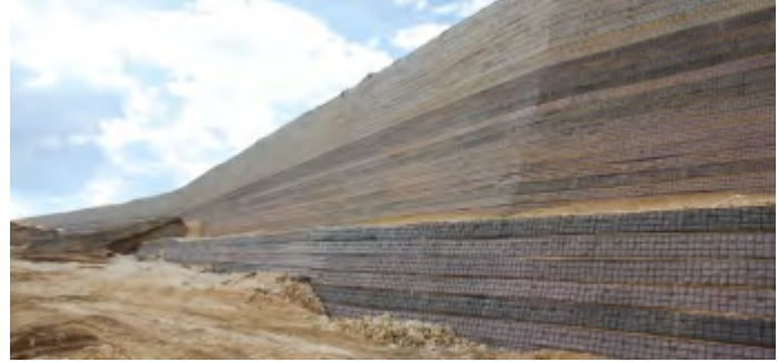
KASTAMONU AIRPORT, PERIPHERAL DRAINAGE AND SLOPE REHABILITATION-TÜRKİYE
