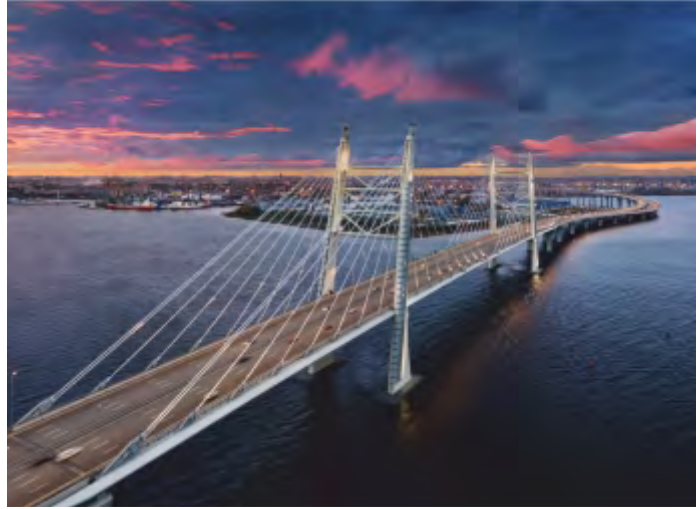
WHSD WESTERN HIGH SPEED DIAMETER MOTORWAY ST. PETERSBURG-THE RUSSIAN FEDERATION
