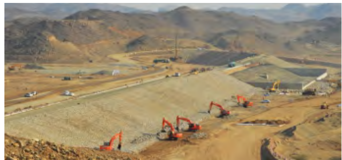
5 DAMS AND SOUTHERN CHANNEL CONSTRUCTION FOR FLOOD PREVENTION (JSDP-2&3) JEDDAH-SAUDI ARABIA
