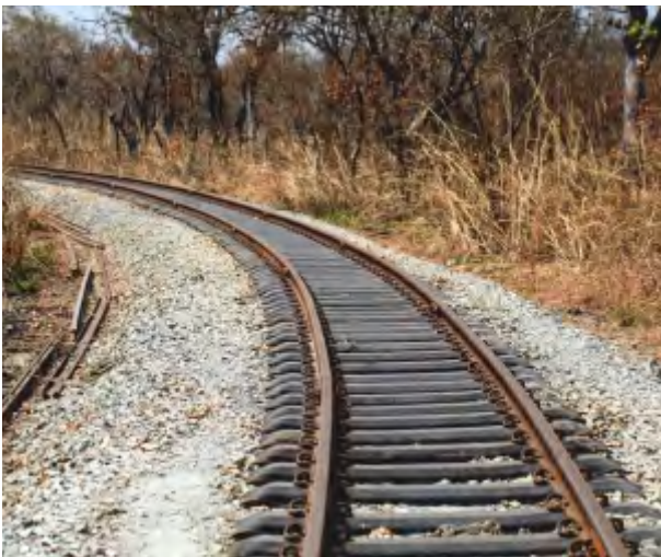
PORT HARCOURT-MAKURDI RAILROAD (463 KM)-NIGERIA
