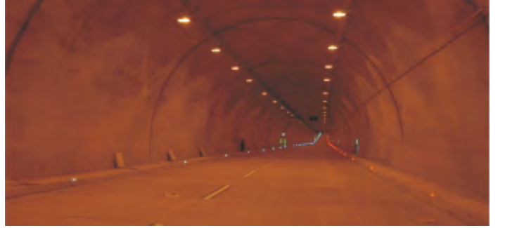
SARIYER-ÇAYIRBAŞI MOTORWAY TUNNEL, İSTANBUL-TÜRKİYE
