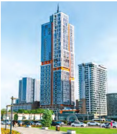
NEST ONE TOWER, TASHKENT-UZBEKISTAN
