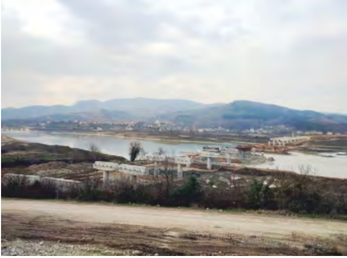
FİLYOS PORT CONNECTION ROADS, BARTIN-TÜRKİYE
