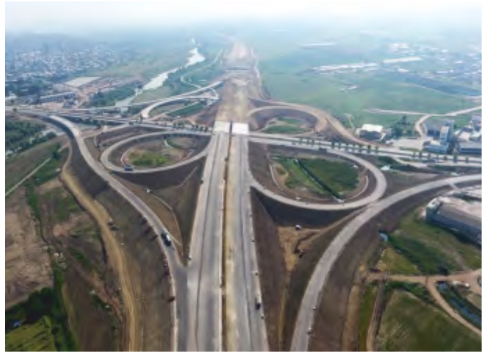
GEBZE-ORHANGAZI MOTORWAY (BURSA-SUSURLUK SECTION)-TÜRKİYE
