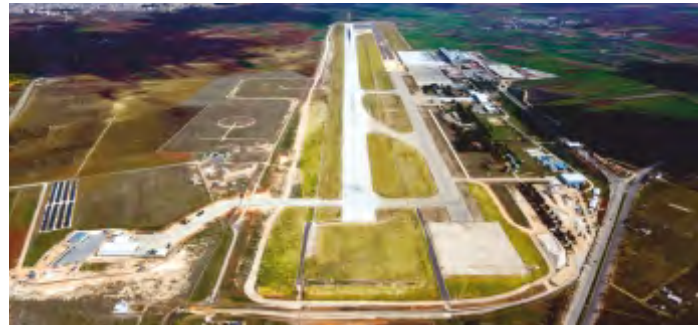
GAZİANTEP AIRPORT, RUNWAY REHABILITATION-TÜRKİYE
