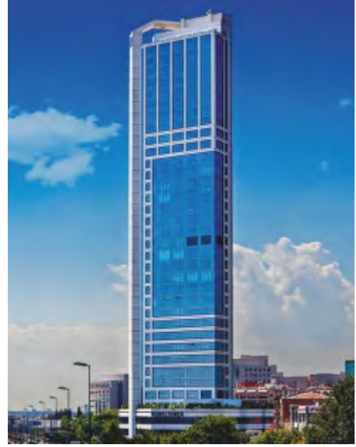
NUROL TOWER ŞTRUCTURAL WORKS (65.000 M2) İSTANBUL-TÜRKİYE
