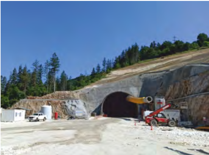
KOSTENEST SEPTEMVRI RAILWAY LINE, PAZARCIK-BULGARIA
