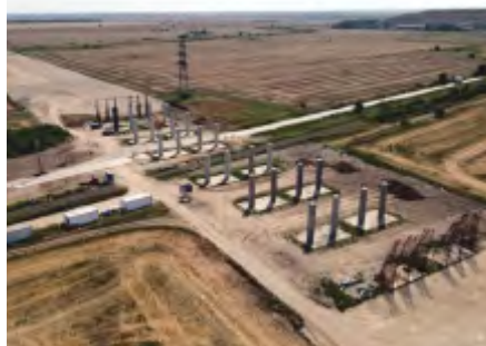
DESIGN AND EXECUTION OF LOT 1 & LOT 2 RING MOTORWAY BUCHAREST-ROMANIA
