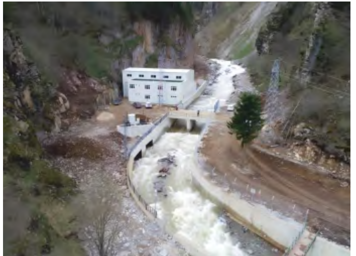
KÖPRÜBAŞI REGULATOR AND HEPP REGULATOR STRUCTURE, GİRESUN-TÜRKİYE
