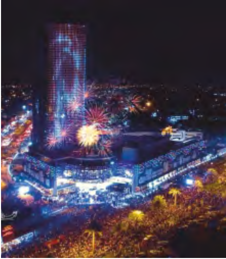
BAGHDAD MALL, HOTEL (5 STAR) AND HOSPITAL COMPLEX IRAQ
