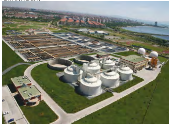
İSKİ ATAĞÖY ADVANCED BIOLOGICAL WASTEWATER TREATMENT PLANT, İSTANBUL-TÜRKİYE
