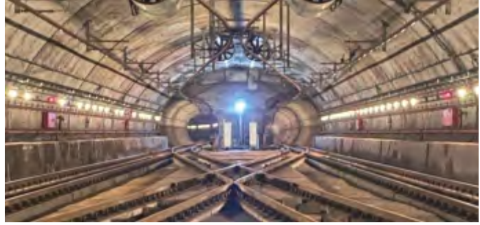
KARTAL-TAVŞANTEPE METRO LINE ELECTRICAL WORKS, İSTANBUL-TÜRKİYE
