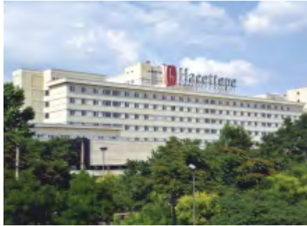
HACETTEPE UNIVERSITY HOSPITAL RENOVATION WORKS ANKARA-TÜRKİYE
