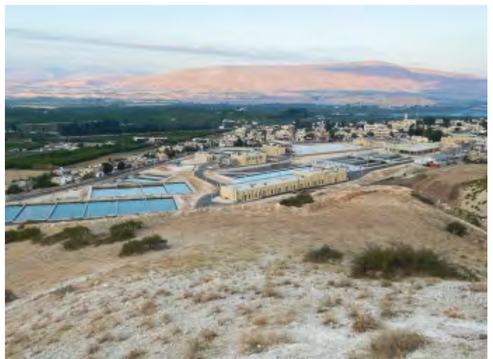
WADI ARAB WATER SYSTEM II (WATER TREATMENT PLANT AND WATER TRANSMISSION PIPELINE)-JORDAN
