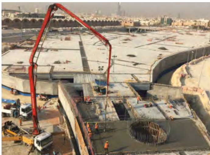
CUT AND COVER TUNNEL STRUCTURAL WORKS AND DEPOT IN LINE 5, RIYADH-SAUDI ARABIA
