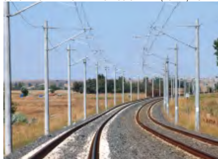
TEKİRDAĞ-MURATLI RAILWAY ELECTRIFICATION-TÜRKİYE
