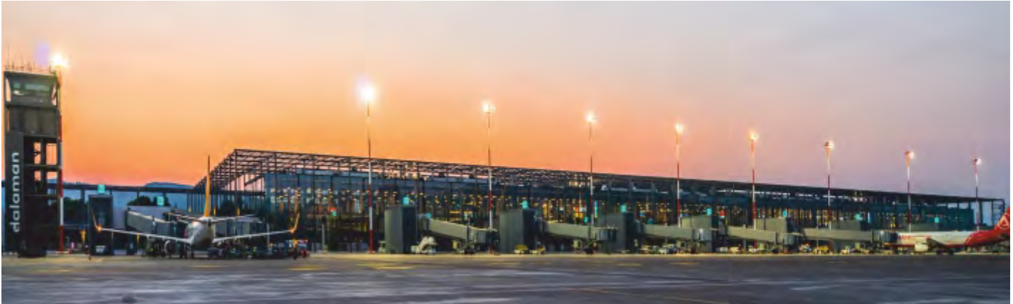
DALAMAN INTERNATIONAL AIRPORT, NEW DOMESTIC AND INTERNATIONAL TERMINAL BUILDING, MUĞLA-TÜRKİYE
