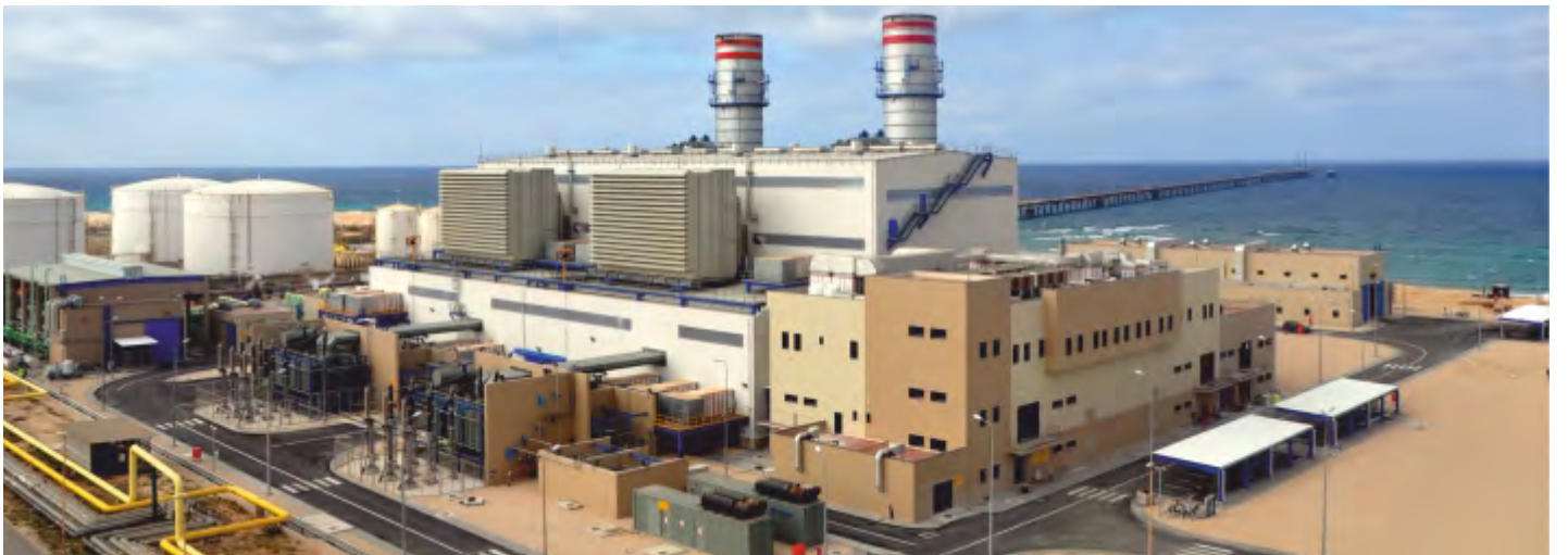
AL-KHUMS FAST TRACK SIMPLE CYCLE POWER PLANT-LIBYA
