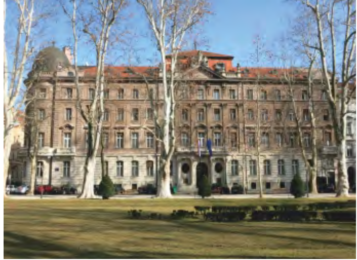
COMPLETE RENOVATION OF THE EARTHQUAKE-DAMAGED BUILDING OF MINISTRY OF FOREIGN AND EUROPEAN AFFAIRS, ZAGREB-CROATIA
