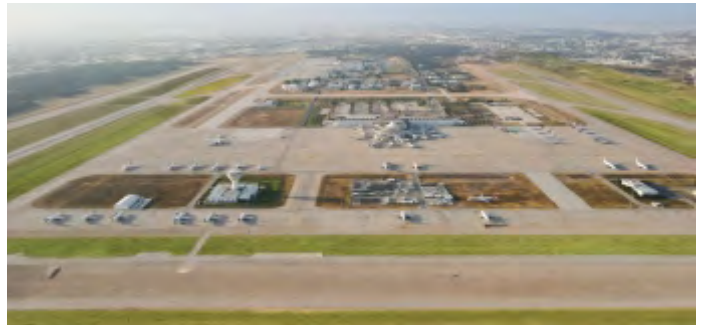
ANTALYA AIRPORT, RUNWAY, TAXIWAY AND APRON REFURBISHMENT-TÜRKİYE
