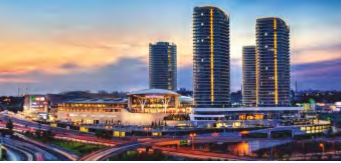
MALL OF İSTANBUL ELECTRICAL WORKS, İSTANBUL-TÜRKİYE
