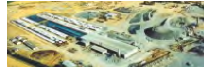
PREFABRICATED CONCRETE ELEMENTS PLANT ŞANLIURFA-TÜRKİYE
