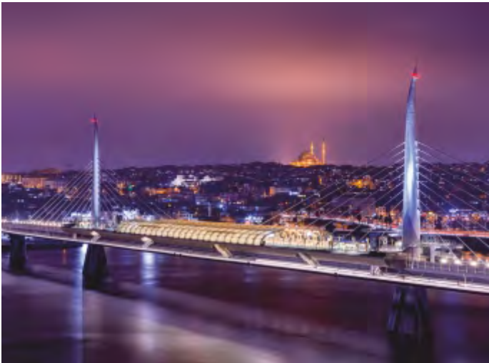
GOLDEN HORN METRO CROSSING BRIDGE, İSTANBUL-TÜRKİYE
