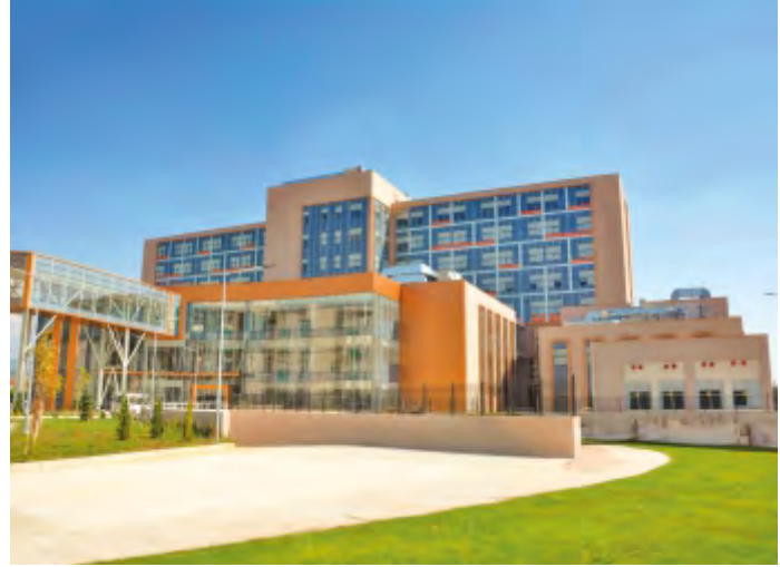
UŞAK STATE HOSPITAL ANNEX BUILDING (200 BEDS), ORAL AND DENTAL HEALTH CENTER (40 UNITS)-TÜRKİYE
