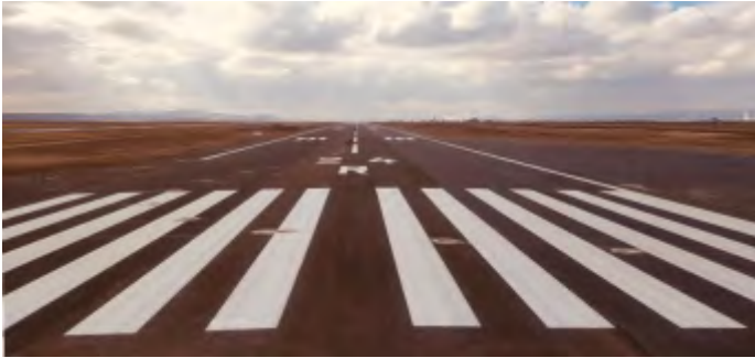
KARS AIRPORT, NEW RUNWAY CONSTRUCTION, APRON AND TAXIWAY REFURBISHMENT-TÜRKİYE
