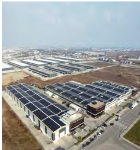
SOLAR POWER PLANT (2280 kW), SAKARYA-TÜRKİYE
