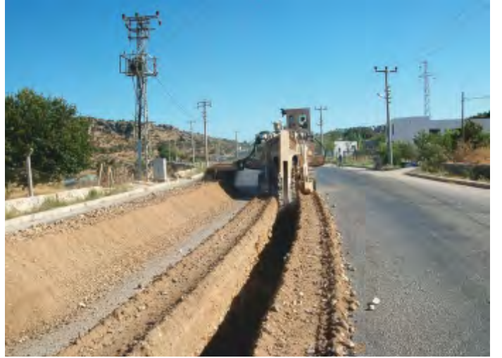
BODRUM EMERGENT WATER SUPPLY, MUĞLA-TÜRKİYE
