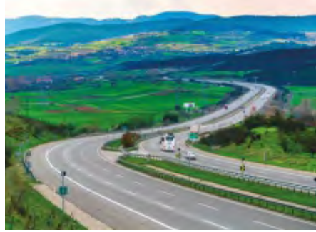
ANATOLIAN HIGHWAY 3rd SECTION INFRASTRUCTURAL WORKS, BOLU-TÜRKİYE
