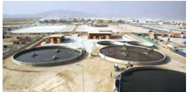
KANDAHAR MILITARY BASE WATER TREATMENT FACILITY-AFGHANISTAN
