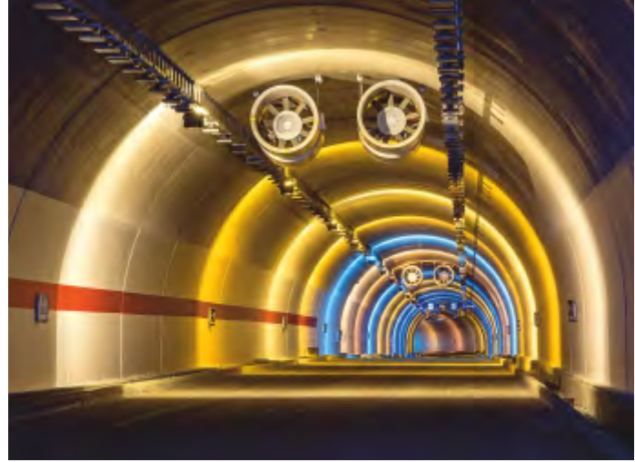
İKİZDERE-İSPİR ROAD, OVİT TUNNEL AND CONNECTION ROADS, RİZE-TÜRKİYE
