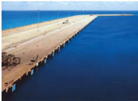
BULK BERTH NO.2, MISURATA-LIBYA
