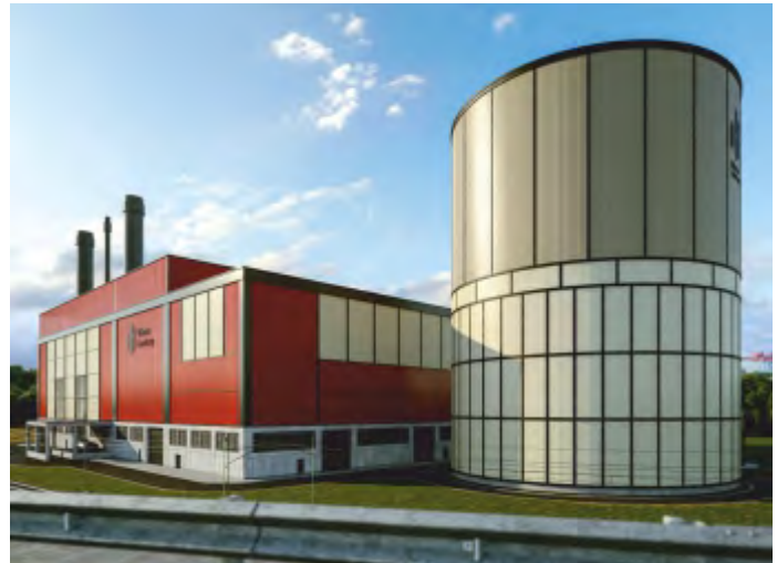
DRADENAU COMBINED HEAT AND POWER PLANT, HAMBURG-GERMANY
