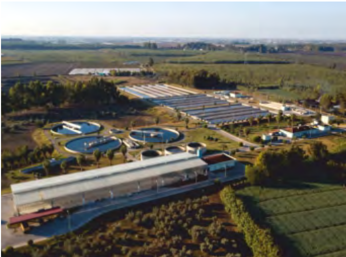
TARSUS WASTE WATER TREATMENT PLANT, MERSİN-TÜRKİYE
