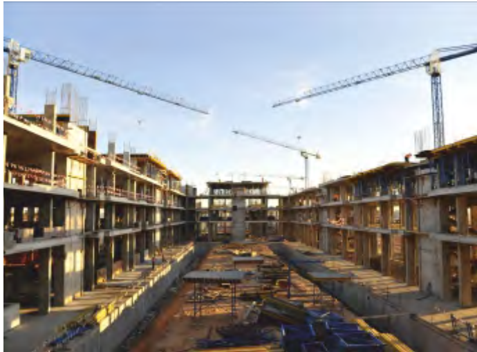
1187 HOUSING UNITS STRUCTURAL WORKS, TRIPOLI-LIBYA
