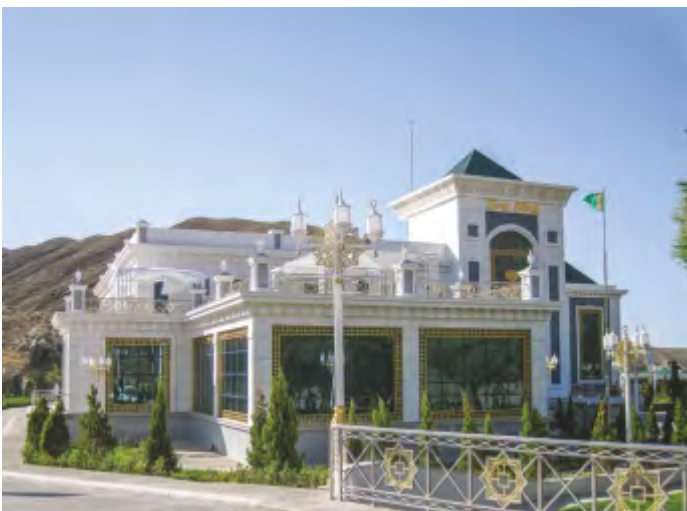
PRESIDENTIAL GUESTHOUSE AND RESTAURANT FACILITIES-TURKMENISTAN
