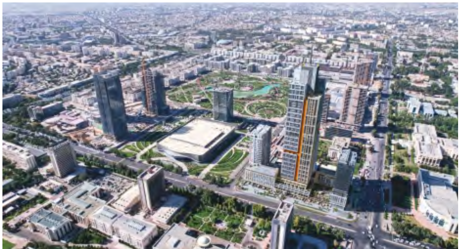
NEST ONE TOWER, TASHKENT-UZBEKISTAN
