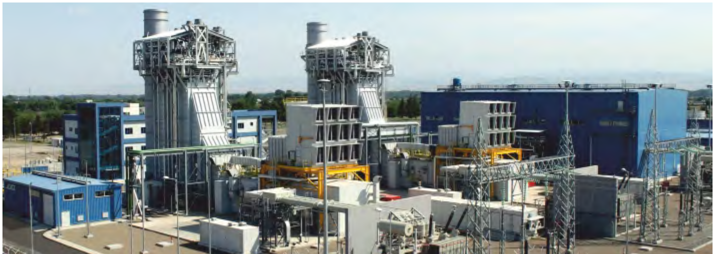
GARDABANI COMBINED CYCLE POWER PLANT-GEORGIA
