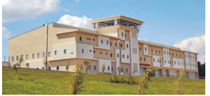
KASTAMONU AIRPORT, FIRE DEPARTMENT AND GARAGE BUILDING CONSTRUCTION-TÜRKİYE
