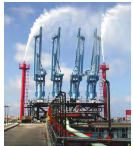
TOBRUK TERMINAL JETTIES-LIBYA
