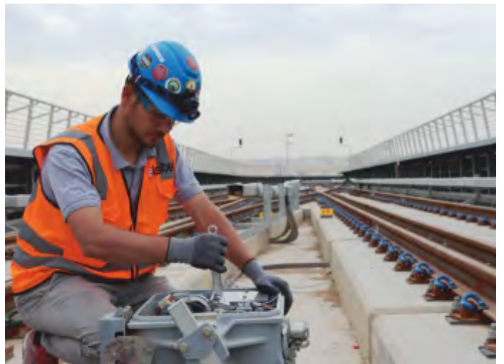
HARAMAIN HIGH SPEED LINE SIGNALING INSTALLATION AND MAINTENANCE WORKS MECCA-MEDINAH-SAUDI ARABIA
