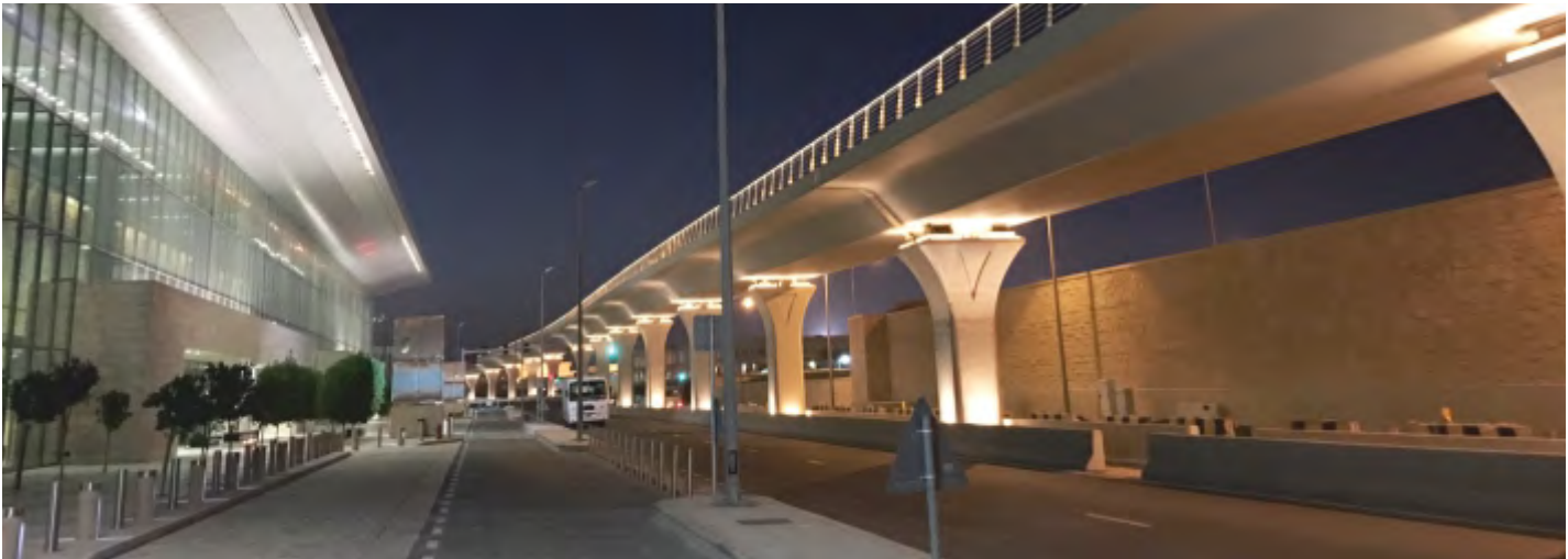
PMS VIADUCT FOR QATAR FOUNDATION, DOHA-QATAR
