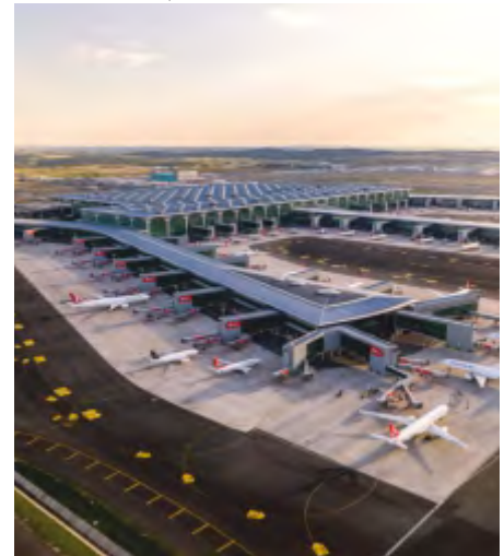
İSTANBUL AIRPORT (PRODUCTION AND INSTALLATION OF DOUBLE TEE FLOORING ELEMENTS)-TÜRKİYE
