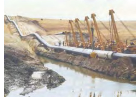
BOTAS ERZURUM-İMRANLI NATURAL GAS PIPELINE ERZURUM-İMRANLI (SİVAS)-TÜRKİYE
