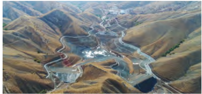
ADIYAMAN WASTE DAM-TÜRKİYE
