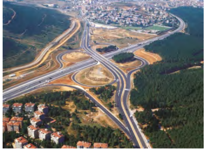
ANADOLU MOTORWAY (CAMLICA-GEBZE SECTION) FRONTAGE HIGHWAYS ORTADAG INTERSECTION, İSTANBUL-TÜRKİYE
