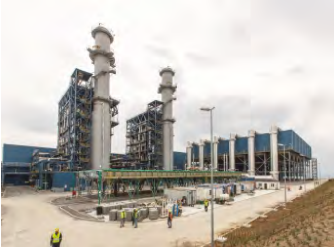
YENİ ELEKTRİK COMBINED CYCLE POWER PLANT (850 MW), KOCAELİ-TÜRKİYE
