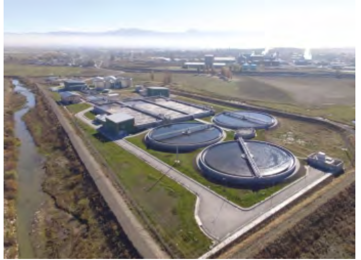
ERZURUM WASTEWATER TREATMENT PLANT-TÜRKİYE
