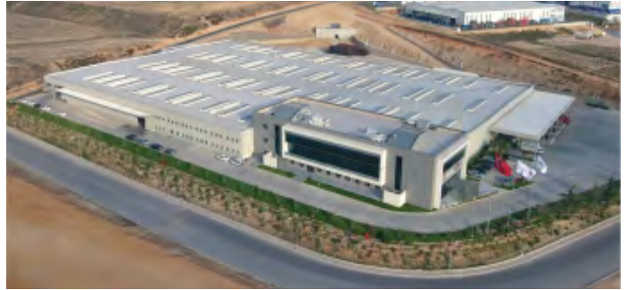
ASKAYNAK (LINCOLN ELECTRIC) FACTORY ELECTRICAL WORKS, KOCAELİ-TÜRKİYE
