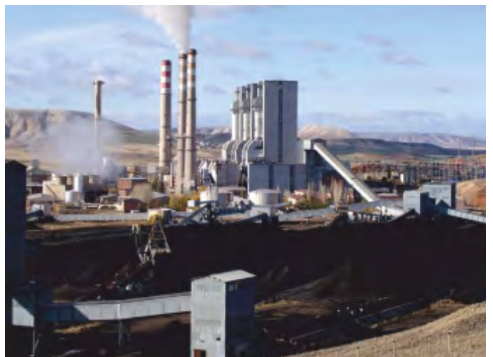
SİVAS KANGAL THERMAL POWER PLANT-TÜRKİYE
