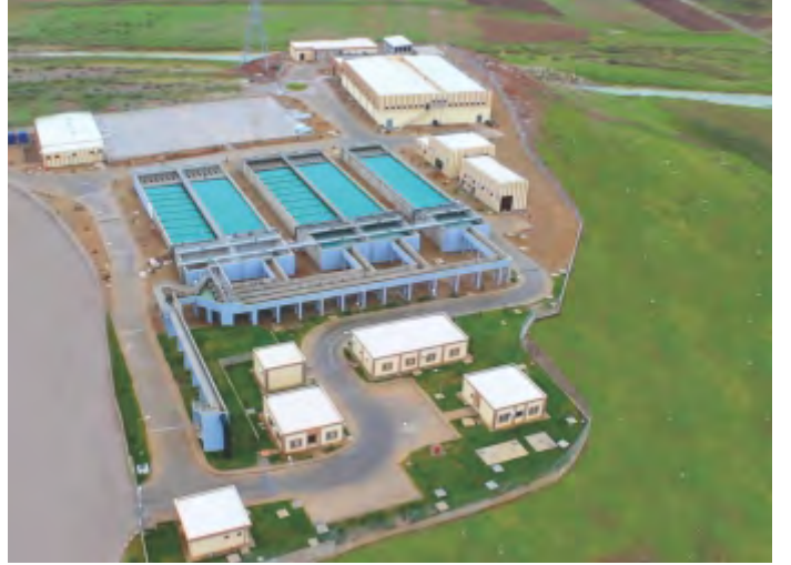
SHAQLAWA SALAHEDIN POTABLE WATER SUPPLY, WATER TREATMENT PLANT AND TRANSMISSION LINES, ERBIL-IRAQ
