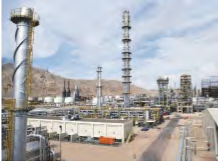
POLYPROPYLENE PLANT, TURKMENBASHI-TURKMENISTAN
