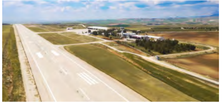
ADIYAMAN AIRPORT, RUNWAY EXTENSION, APRON AND TAXIWAY REFURBISHMENT-TÜRKİYE
