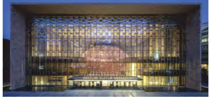
ATATÜRK CULTURAL CENTER ELECTRICAL WORKS, İSTANBUL-TÜRKİYE
