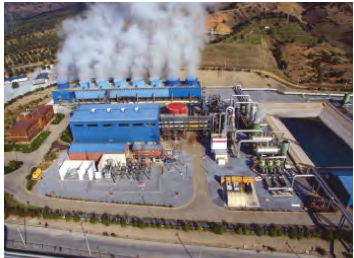
GALİP HOCA GEOTHERMAL POWER PLANT, ADIN-TÜRKİYE
