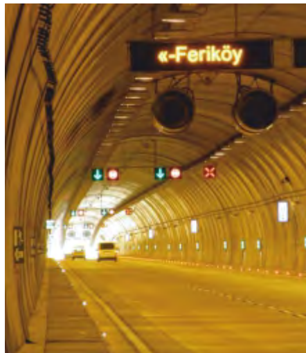
DOLMABAÇE-DOLAPDERE-KAĞITHANE-PIYALEPAŞA TUNNELS, İSTANBUL-TÜRKİYE
