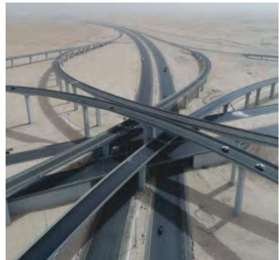
RA 245-ROADS AND INTERCHANGES CONSTRUCTION, UPDAGING AND MAINTENANCE, MUTLAA CITY-KUVEYT
