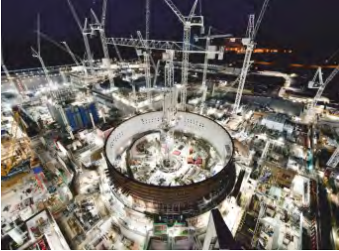
HINKLEY POINT C (HPC) NUCLEAR POWER PLANT TURBINE ISLAND HP AND IP/LP PIPING PREFABRICATION AND ERECTION WORKS, BRIDGWATER, SOMERSET-THE UNITED KINGDOM
