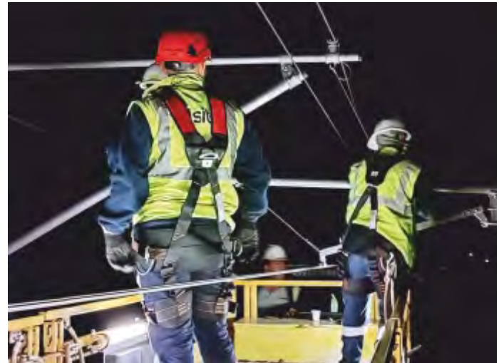
POLATLI-KONYA HIGH SPEED LINE ELECTRIFICATION MAINTENANCE, POLATLI-KONYA-TÜRKİYE
