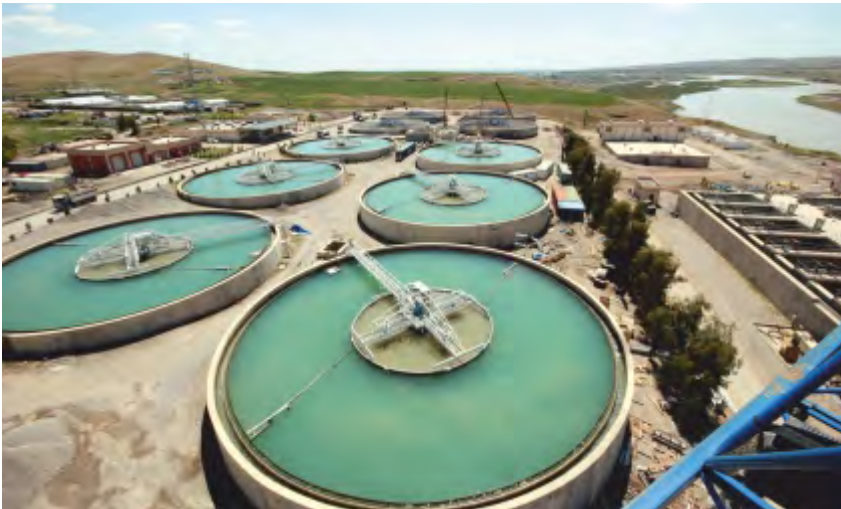
ERBIL WATER TREATMENT FACILITY AND SUPPLY NETWORK-IRAQ
