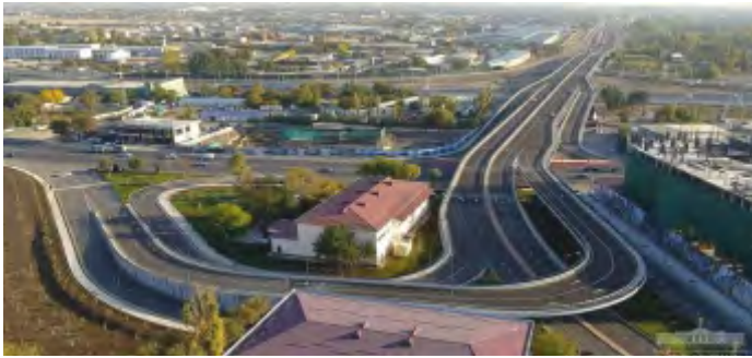
ROAD AND BRIDGE, TASHKENT-UZBEKISTAN
