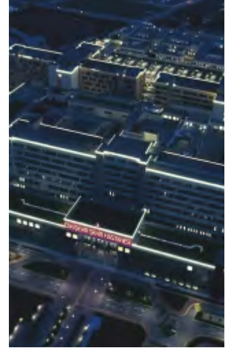
ESKİŞEHİR CITY HOSPITAL-TÜRKİYE
