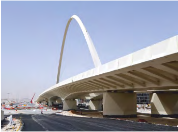
LUSAIL DEVELOPMENT INFRASTRUCTURE PACKAGE 4, DOHA-QATAR
