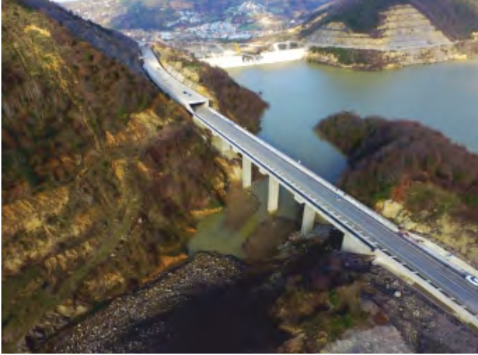
KİRAZLIKÖPRÜ DAM ROAD, BARTIN-TÜRKİYE
