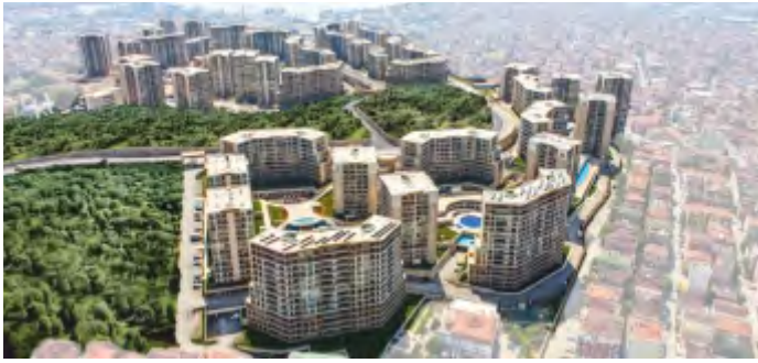
EVORA İSTANBUL ELECTRICAL WORKS, İSTANBUL-TÜRKİYE
