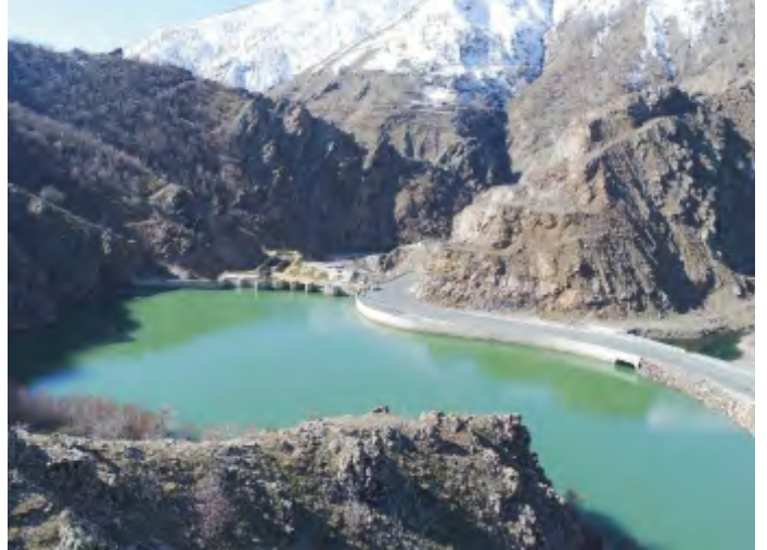
KULP1 AND KULP4 HYDROELECTRIC POWER PLANT, DİYARBAKIR-TÜRKİYE
