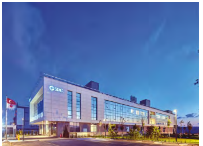
SMC OFFICE AND FACTORY BUILDING, İSTANBUL-TÜRKİYE
