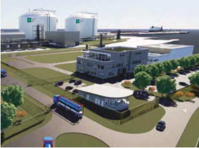
STADE LIQUEFIED NATURAL GAS (LNG) REGASIFICATION TERMINAL, STADE-GERMANY
