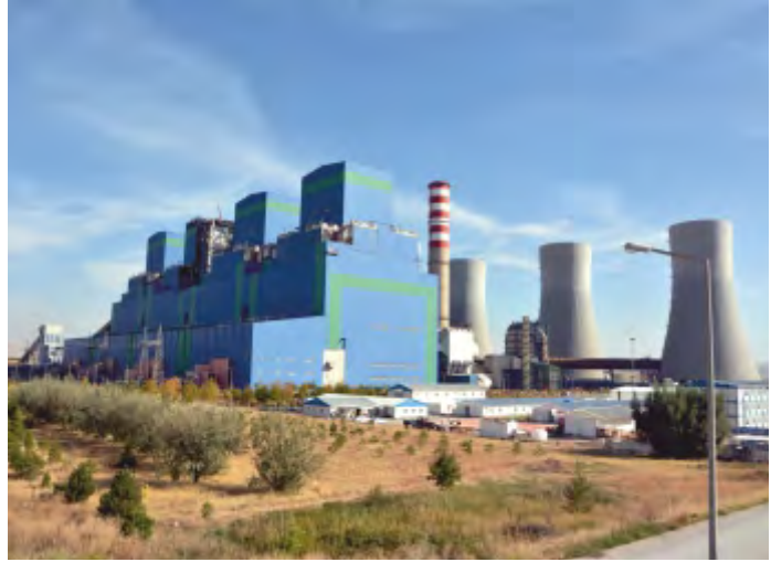
AFSİN-ELBİSTAN B THERMAL POWER PLANT UNIT 2 REHABILITATION KAHRAMANMARAŞ-TÜRKİYE
