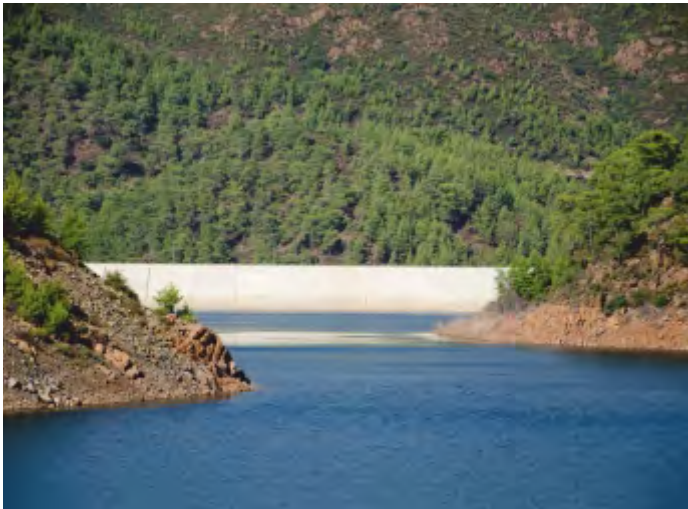
MARMARİS POTABLE WATER DAM, MUĞLA-TÜRKİYE
