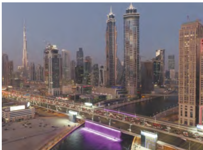
DUBAI WATER CANAL SHEIKH ZAYED ROAD BRIDGE CROSSING-UAE
