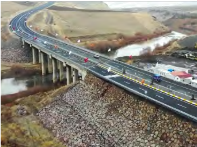
ROAD AND BRIDGE, AĞRI-TÜRKİYE
