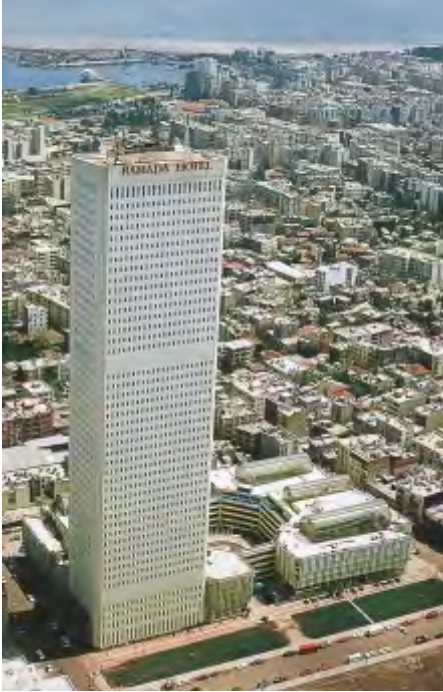
MERSİN METROPOL HIGH RISE BUILDING-TÜRKİYE
