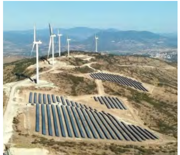
ÇAYPINAR 2 WEPP (24 MW) AND ÇAYPINAR SOLAR POWER PLANT (5,5 MW) BALIKESİR-TÜRKİYE
