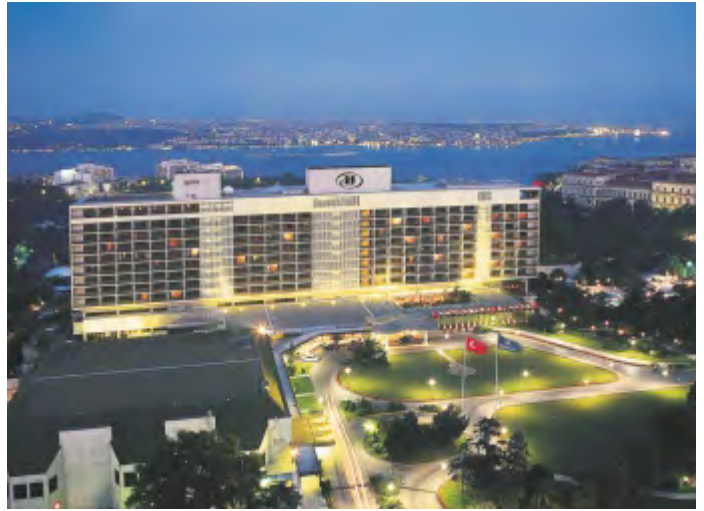
HILTON HOTEL EARTHQUAKE REINFORCEMENT AND MODERNIZATION, İSTANBUL-TÜRKİYE
