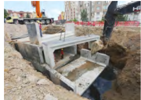
İSKİ 7TH DISTRICT WASTEWATER, RAIN WATER CANAL AND RIVER RECLAMATION, İSTANBUL-TÜRKİYE
