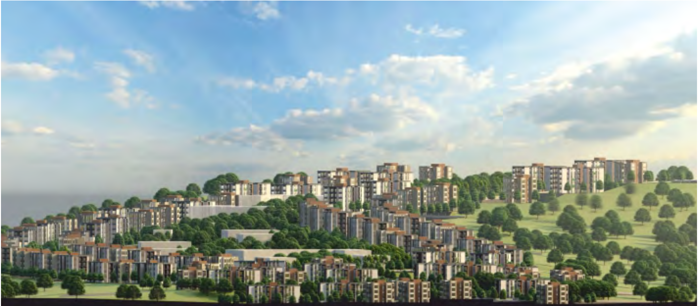
1502 RESIDENCE AND LANDSCAPE WORKS, ANTAKYA, HATAY-TÜRKİYE
