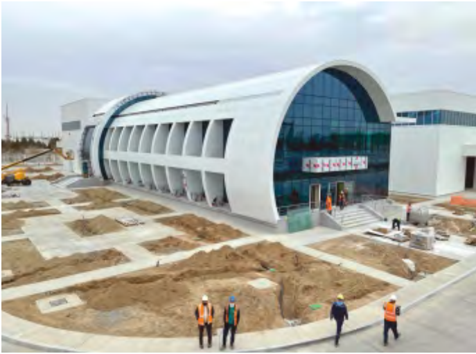
SERVICE AND MAINTENANCE CENTER-TURKMENISTAN
