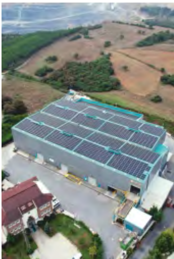
SOLAR POWER PLANT (800 kW) KOCAELİ-TÜRKİYE
