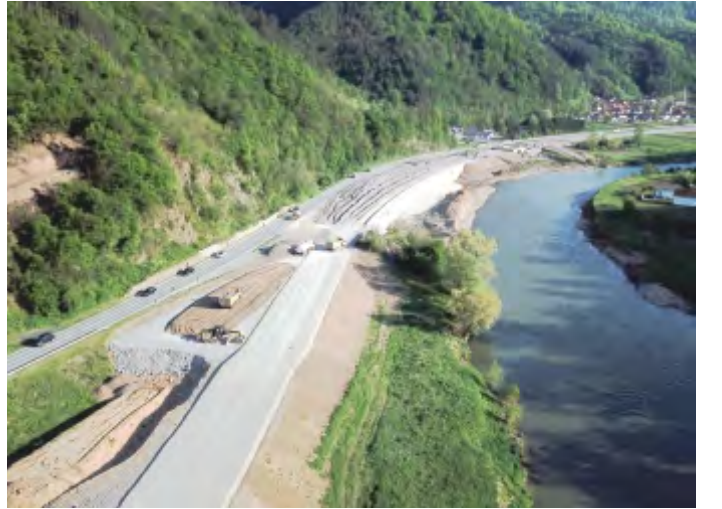
MOTORWAY ON CORRIDOR VC., SECTION NEMİLA-VRANDUK-BOSNIA HERZEGOVINA
