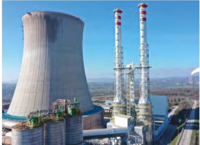
18MART ÇAN FLUE GAS DESULPHURISATION PLANT (2X160 MW), ÇANAKKALE-TÜRKİYE
