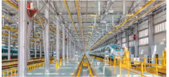
ANKARA HIGH SPEED TRAIN DEPOT AND MAINTENANCE COMPLEX-TÜRKİYE
