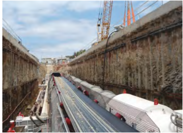
CASABLANCA CITY FLOOD PROTECTION TUNNEL-MOROCCO
