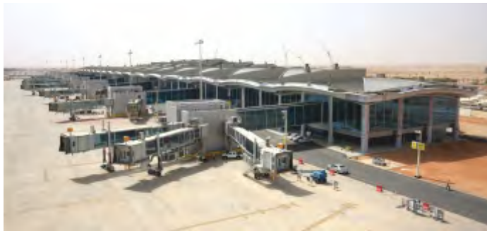
RIYADH KING KHALED AIRPORT TERMINAL 5-SAUDI ARABIA
