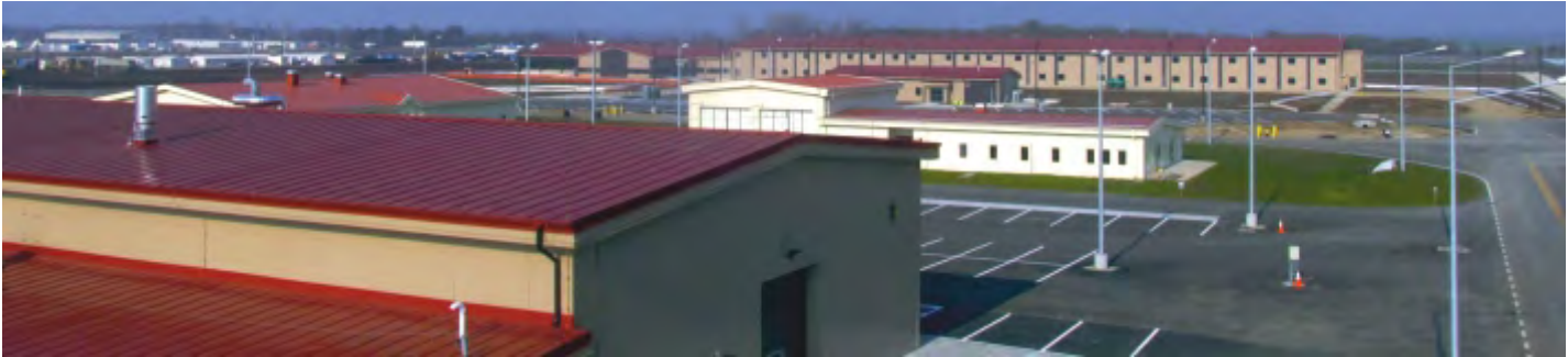
EUROPEAN MILITARY SUPPORT FACILITIES PHASE II, DEVESELU-ROMANIA
