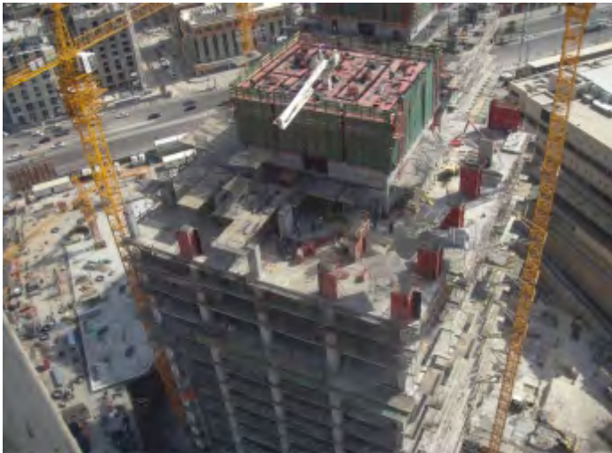
OLAYA TOWERS, RIYADH-SAUDI ARABIA
