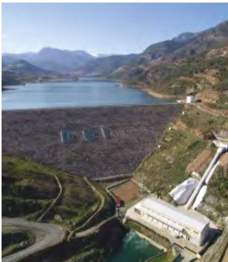
MESA PROJE ALAKÖPRÜ DAM AND HEPP, MERSİN-TÜRKİYE
