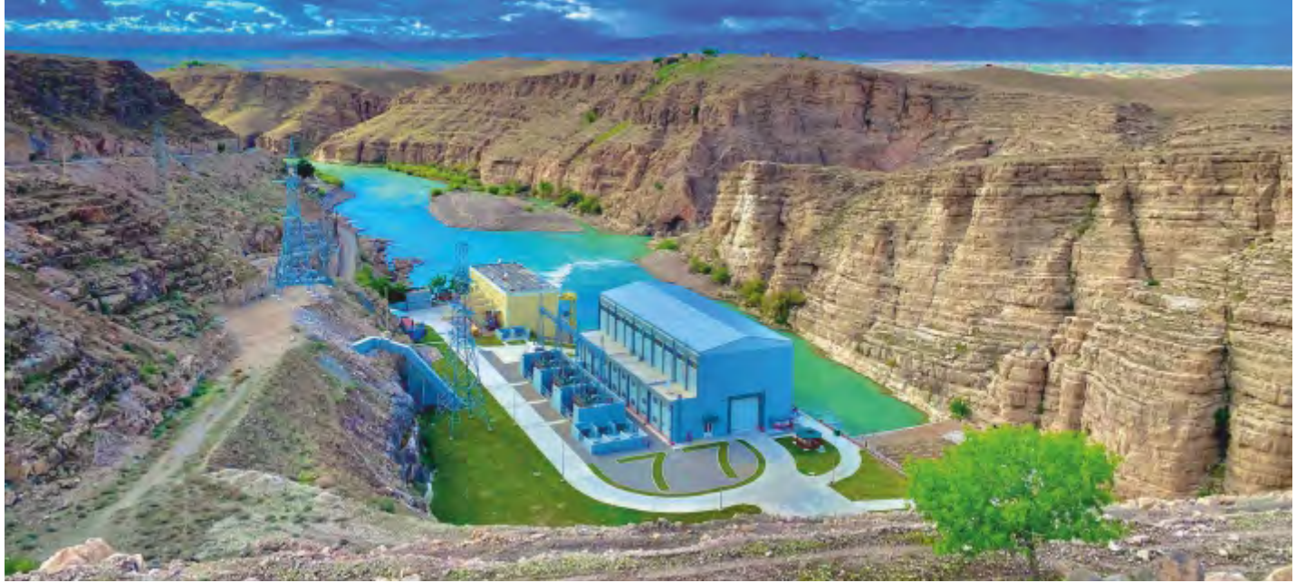
KAJAKI DAM (100 MW) EXPENSION-AFGHANISTAN
