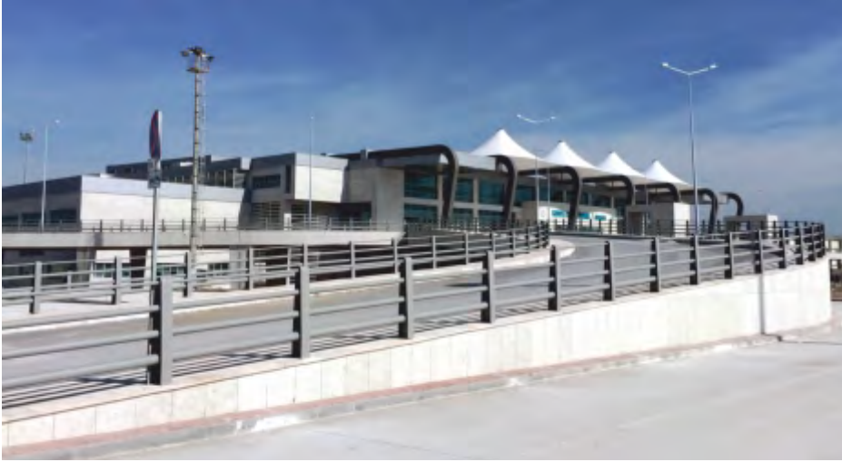
KONYA AIRPORT TERMINAL BUILDING, KONYA-TÜRKİYE
