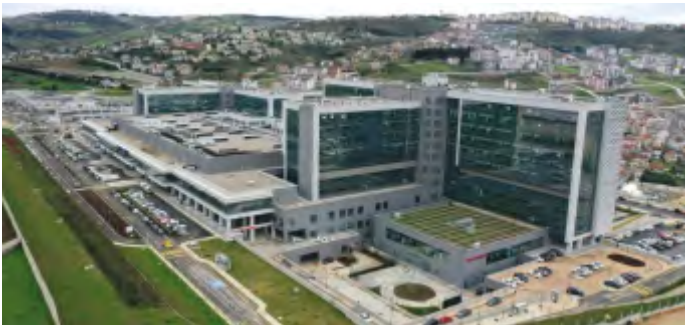
KOCAELİ INTEGRATED HEALTHCARE CAMPUS ELECTRICAL WORKS, KOCAELİ-TÜRKİYE
