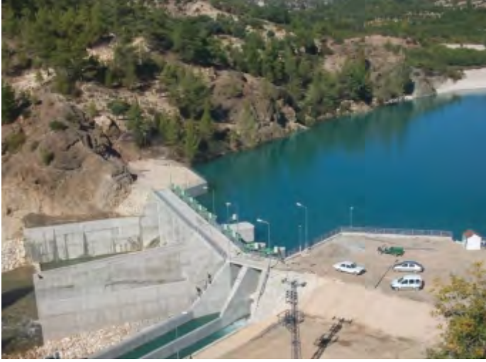
SARIKAVAK HYDROELECTRIC POWER PLANT, MERSİN-TÜRKİYE
