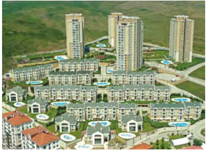
UPHILL COURT BAĞÇEŞEHİR, İSTANBUL-TÜRKİYE
