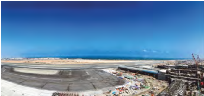
MUSCAT AIRPORT INFRASTRUCTURE WORKS-OMAN
