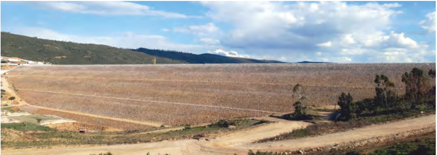
BOUKHROUFA DAM, TARF-ALGERIA
