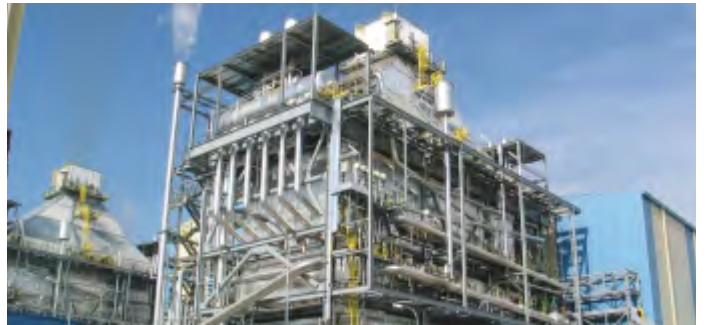
TEMLİ NİĞAL GAS COMBİED CYCLE POWER PLANT, ANKARA-TÜRKİYE
