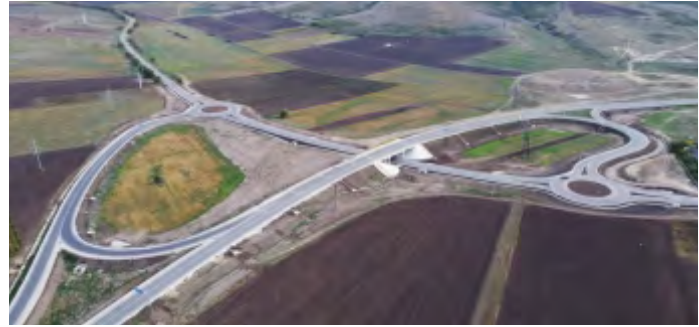
COMRAT BYPASS ROAD (M-3) CEADİR-LUNGA INTERCHANGE-MOLDOVA
