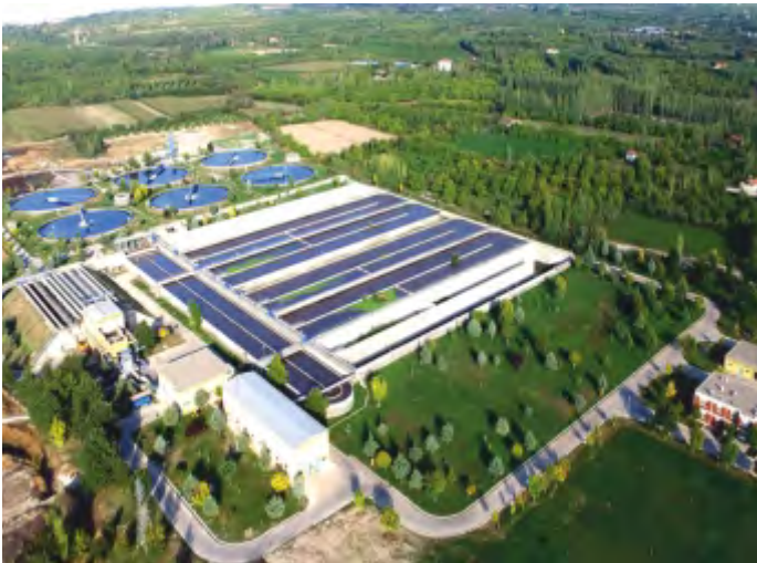
ŞANLIURFA POTABLE WATER SEVERAGE PLANT-TÜRKİYE
