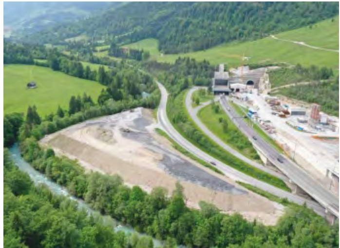
KARAVANKE HIGHWAY TUNNEL-SLOVENIA
