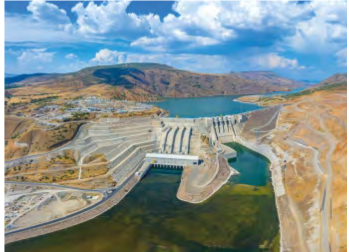
LOWER KALEKÖY DAM AND HEPP (500 MW-1193 GWh), BİNGÖL-TÜRKİYE
