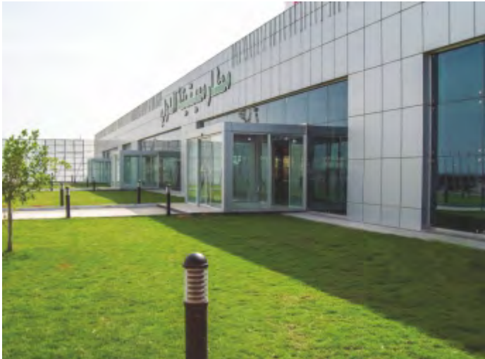
MITIGA AIRPORT'S VIP LOUNGE, TRIPOLI-LIBYA
