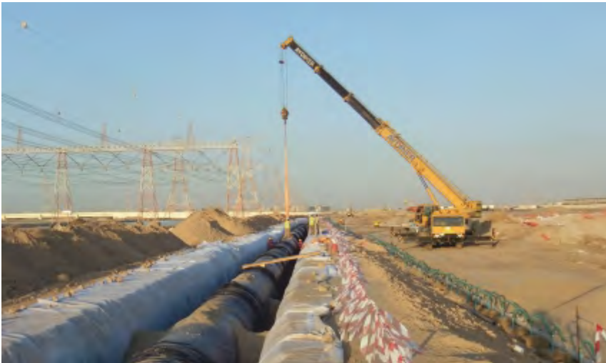
MUSSAFAH-ABU DHABI WATER SUPPLY PROJECT-UAE
