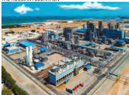
SOCAR POLYMER POLYETHYLENE PLANT SUMQAYIT-AZERBAIJAN
