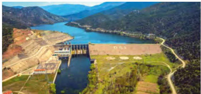
YENİCE DAM AND HEPP, ESKİŞEHİR-TÜRKİYE
