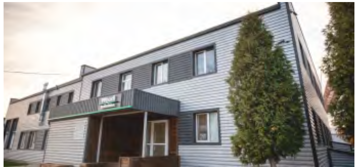
WOOD INDUSTRIES MANAGEMENT BUILDING, LVIV-UKRAINE
