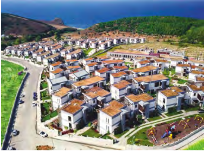
EPP THERMAL CITY 413 UNITS OF HOUSING, YALOVA-TÜRKİYE
