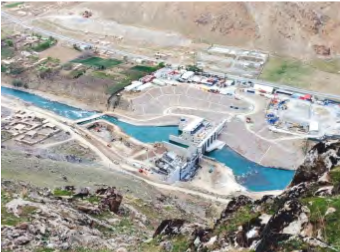
FAIZABAD DAM AND HYDROPOWER PLANT-AFGHANISTAN
