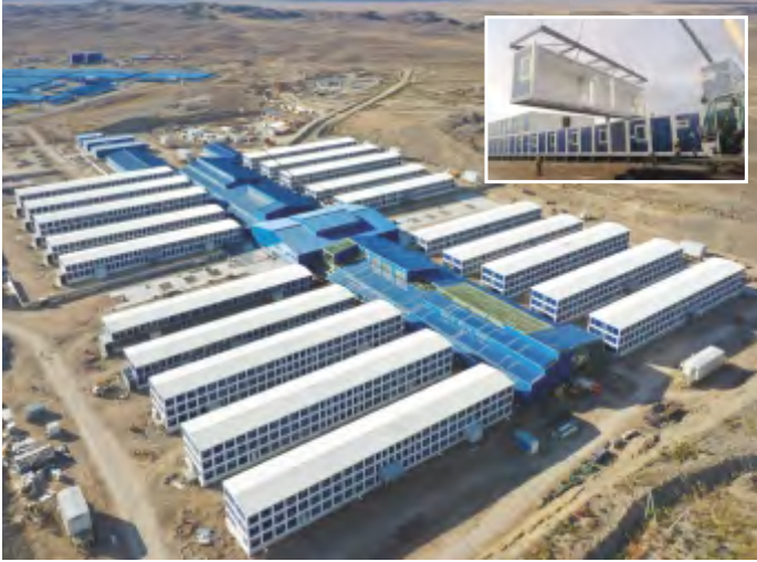
AKTOGAY COPPER MINING EXPANSION PROJECT WORKER ACCOMMODATION CAMP (FOR 2.700 MAN), AKTOGAY-KAZAKHSTAN
