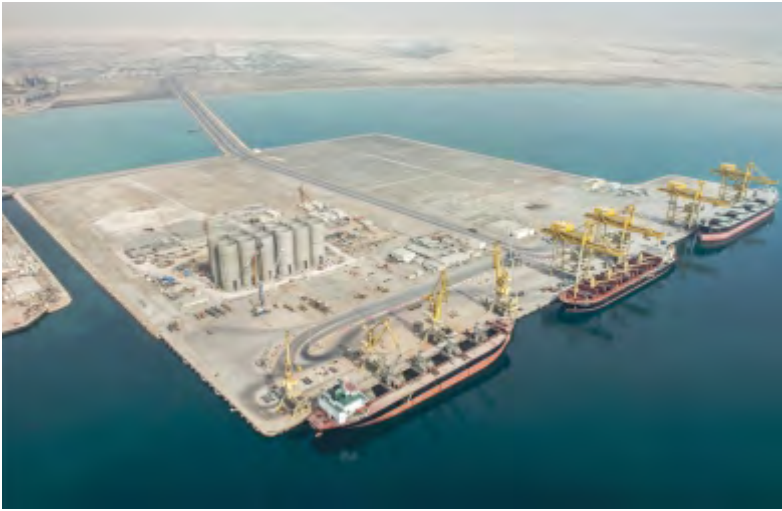
EPIC FOR GABBRO BERTH EXPANSION-QATAR
