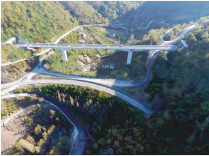
VIADUCT AND TUNNEL, ZONGULDAK-TÜRKİYE
