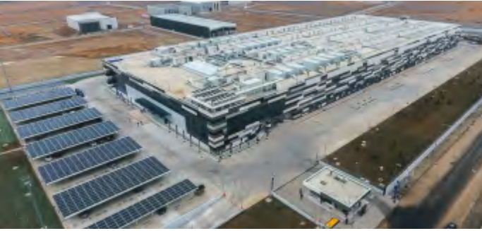
TURKCELL DATA CENTER ELECTRICAL WORKS, ANKARA/KOCAELİ-TÜRKİYE
