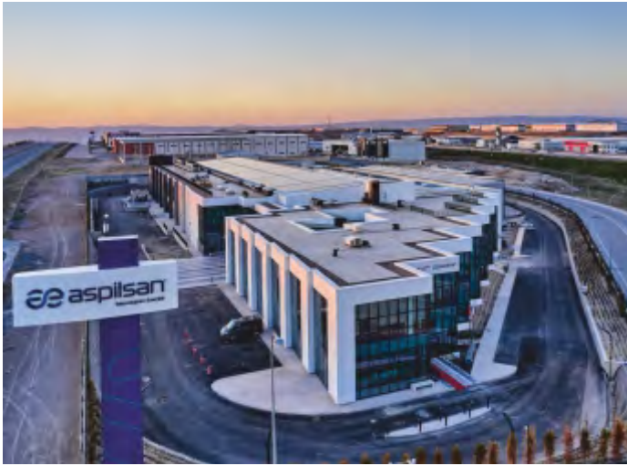
ASPILSAN LITHIUM ION BATTERY PLANT, KAYSERİ-TÜRKİYE
