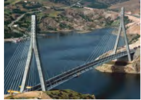
NISSİBİ CABLE STAYED BRIDGE, ADIYAMAN-TÜRKİYE
