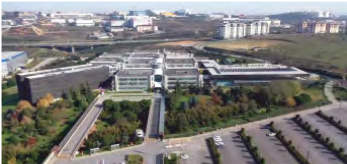
YAPI KREDİ BANKING CENTER ELECTRICAL WORKS, KOCAELİ-TÜRKİYE
