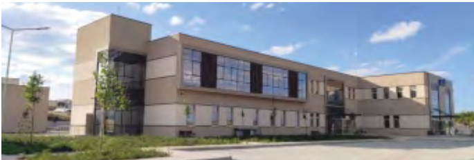
BURDUR PROVINCIAL EMERGENCY DISASTER MANAGEMENT CENTER BUILDING-TÜRKİYE
