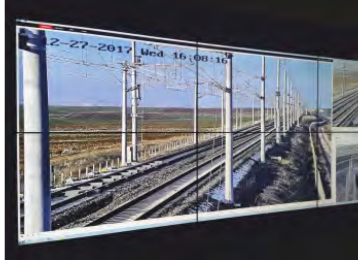
POLATLI-KONYA HIGH SPEED LINE CCTV SYSTEMS, POLATLI-KONYA-TÜRKİYE
