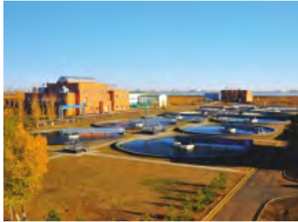
TALDYKOL SEWER POND LIQUIDATION PHASE 1-2-3-4-5 TALDYKOL-KAZAKHSTAN
