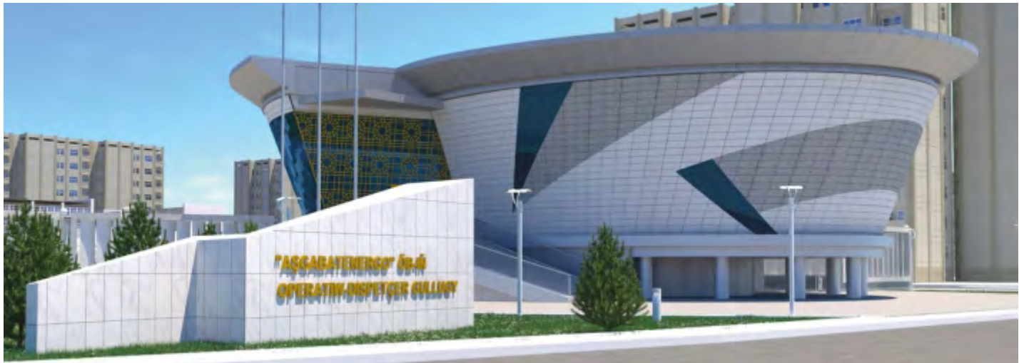
URBAN ENERGY INFRASTRUCTURE REINFORCEMENT PROJECT, ASHGABAT-TURKMENISTAN
