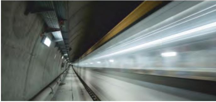
YENİ HAVALİMANI-HALKALI METRO LINE ELECTRICAL WORKS, İSTANBUL-TÜRKİYE
