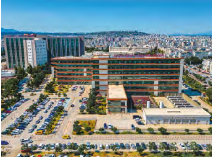
ANTALYA EDUCATION AND RESEARCH HOSPITAL ADDITIONAL BUILDING (300 BEDS) OBSTETRICS AND GYNECOLOGY HOSPITAL-TÜRKİYE
