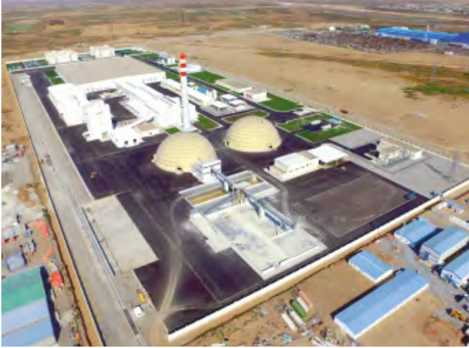
FLAT GLASS AND CONTAINER GLASS PLANT, ASHGABAT-TURKMENISTAN
