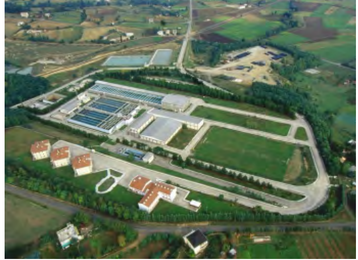
SAMSUN POTABLE WATER TREATMENT PLANT-TÜRKİYE
