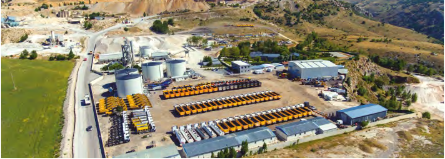
KIBRISKÖY ASPHALT, MASTIC ASPHALT AND EMULSION PRODUCTION PLANT, ANKARA-TÜRKİYE
