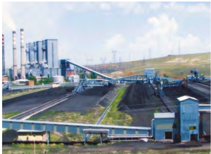
KANGAL THERMAL POWER PLANT, SİVAS-TÜRKİYE
