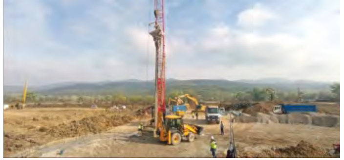
SAGAREJO RINGROAD CONSTRUCTION WORKS (LOT 2)-GEORGIA
