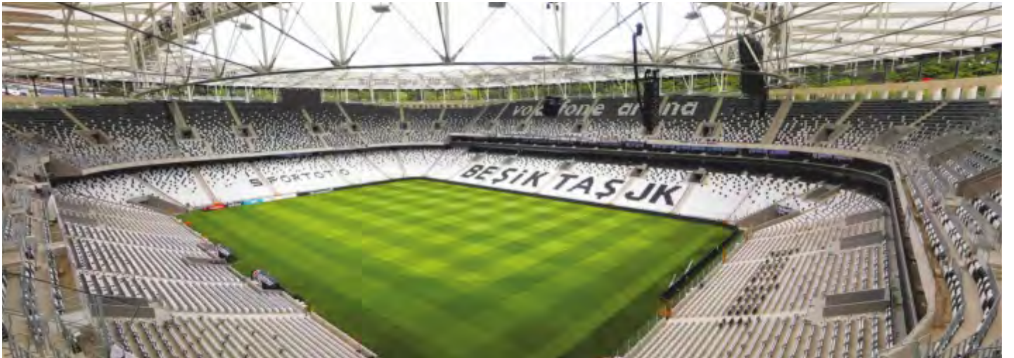
BEŞİKTAŞ VODAFONE ARENA STADIUM PRECAST STAND STEPS, İSTANBUL-TÜRKİYE
