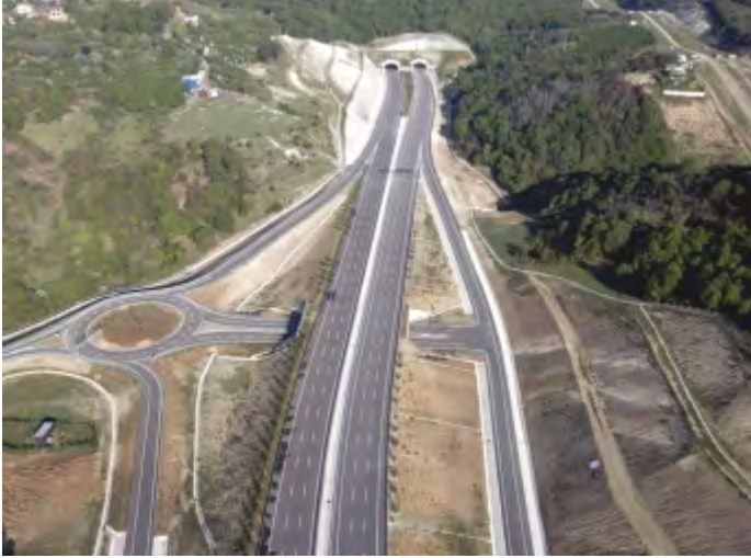
ŞİLE-AĞVA CONNECTION ROAD, İSTANBUL-TÜRKİYE
