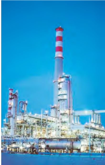
DIESEL KEROSENE HYDR PROCESS AND CCR REFORMER KIRIKKALE-TÜRKİYE
