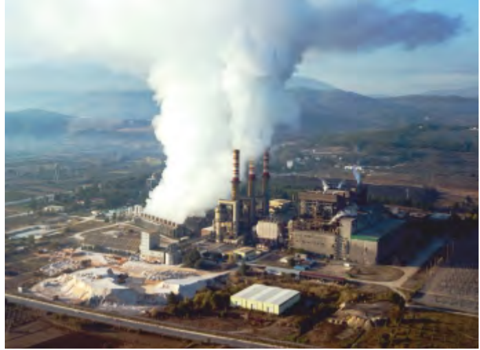
YATAĞAN TPP, FLUE GAS DESULPHURIZATION UNIT, MUĞLA-TÜRKİYE
