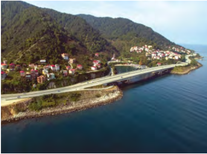
GÜLBURNU BRIDGE, GİRESUN-ESPIYE HIGHWAY-TÜRKİYE
