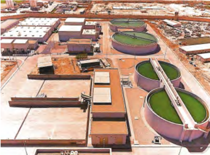
BESMAYAH WATER TREATMENT, BAGHDAD-IRAQ
