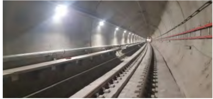
DUDULLU-BOSTANCI METRO LINE ELECTRICAL WORKS, İSTANBUL-TÜRKİYE
